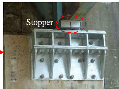
Application of steel bracket with unseating prevention stopper
