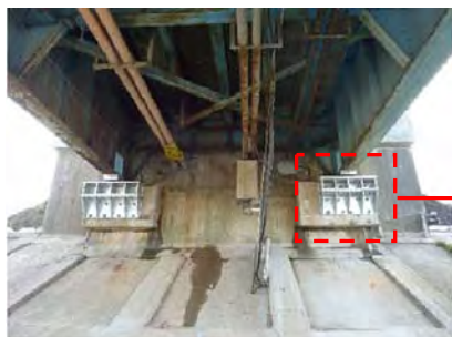
Application of steel bracket with unseating prevention stopper
