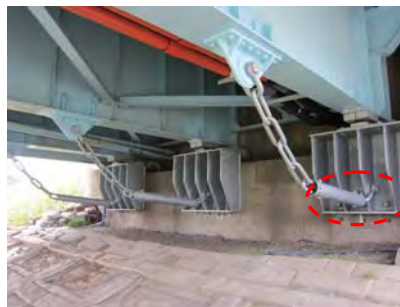
Application of steel bracket with unseating prevention chain
