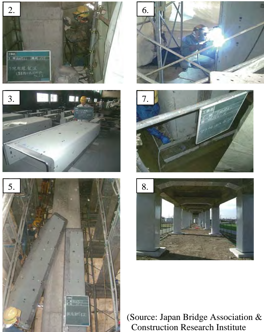
Figure 3.2.2-1 Construction Steps of Steel Plate Jacketing
