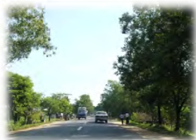
Road No.2 (radial road)
