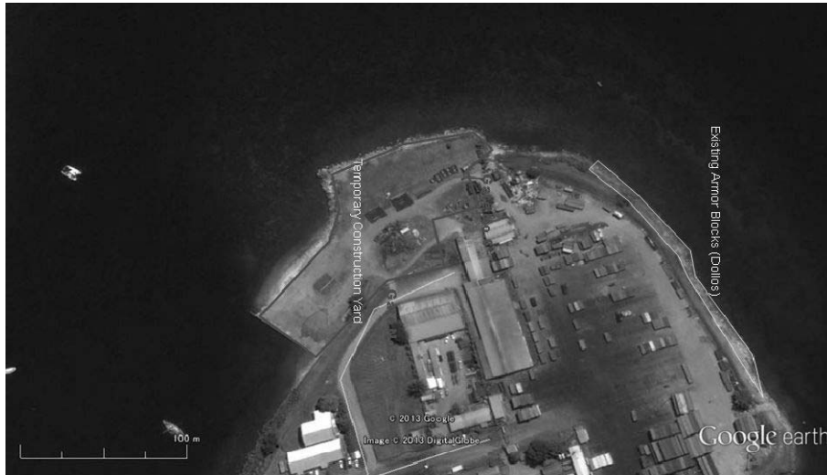
Figure 2.2.4.1-1 Location of Temporary Construction Yard
