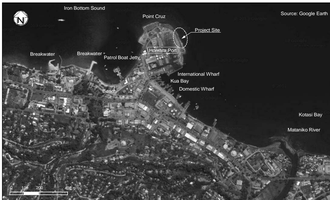
Figure 2.2.2.1-22 Coastal Structures around the Project Site
