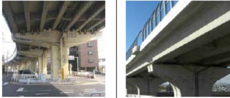
Figure 3-14 Images of Precast Box Girder bridges
