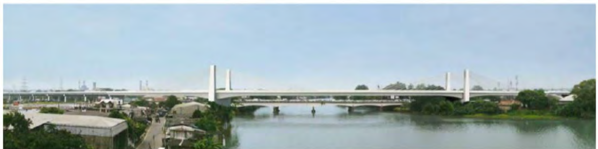
Figure 3-13 Main bridge across Kelani River (Extra dosed type bridge)
