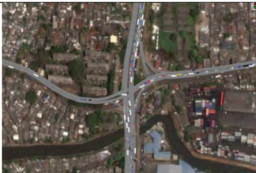
Orugudawatta Intersection (Current)
