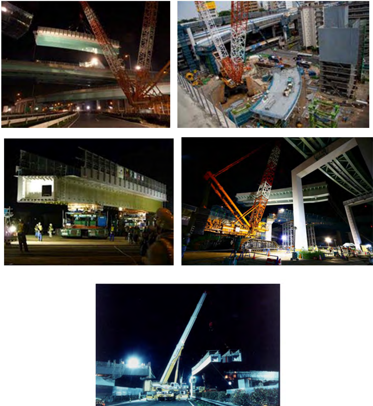
Figure 5.2.39 Some Examples of Girder Erection Work
