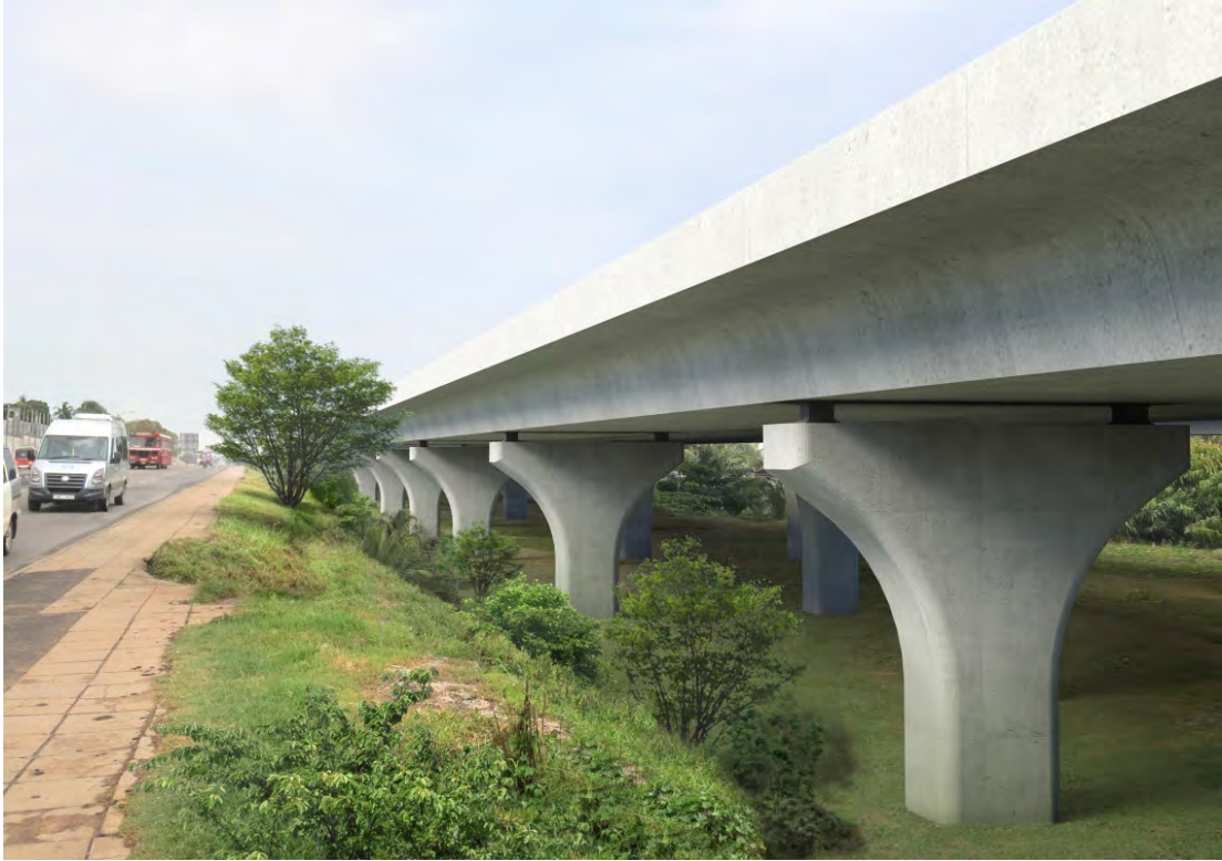
View of Approach Bridge of PC Box Girder from Existing Road
