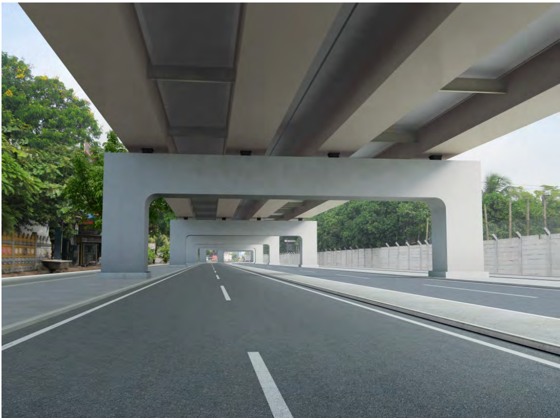
View of Approach Bridge of Steel Box Girder from Existing Road
