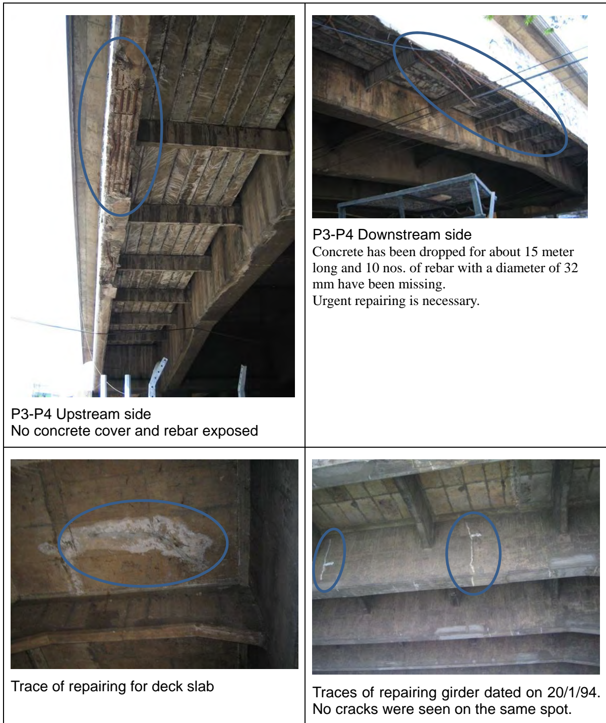
Figure 2.4.2 Bridge Conditions (1/2)
