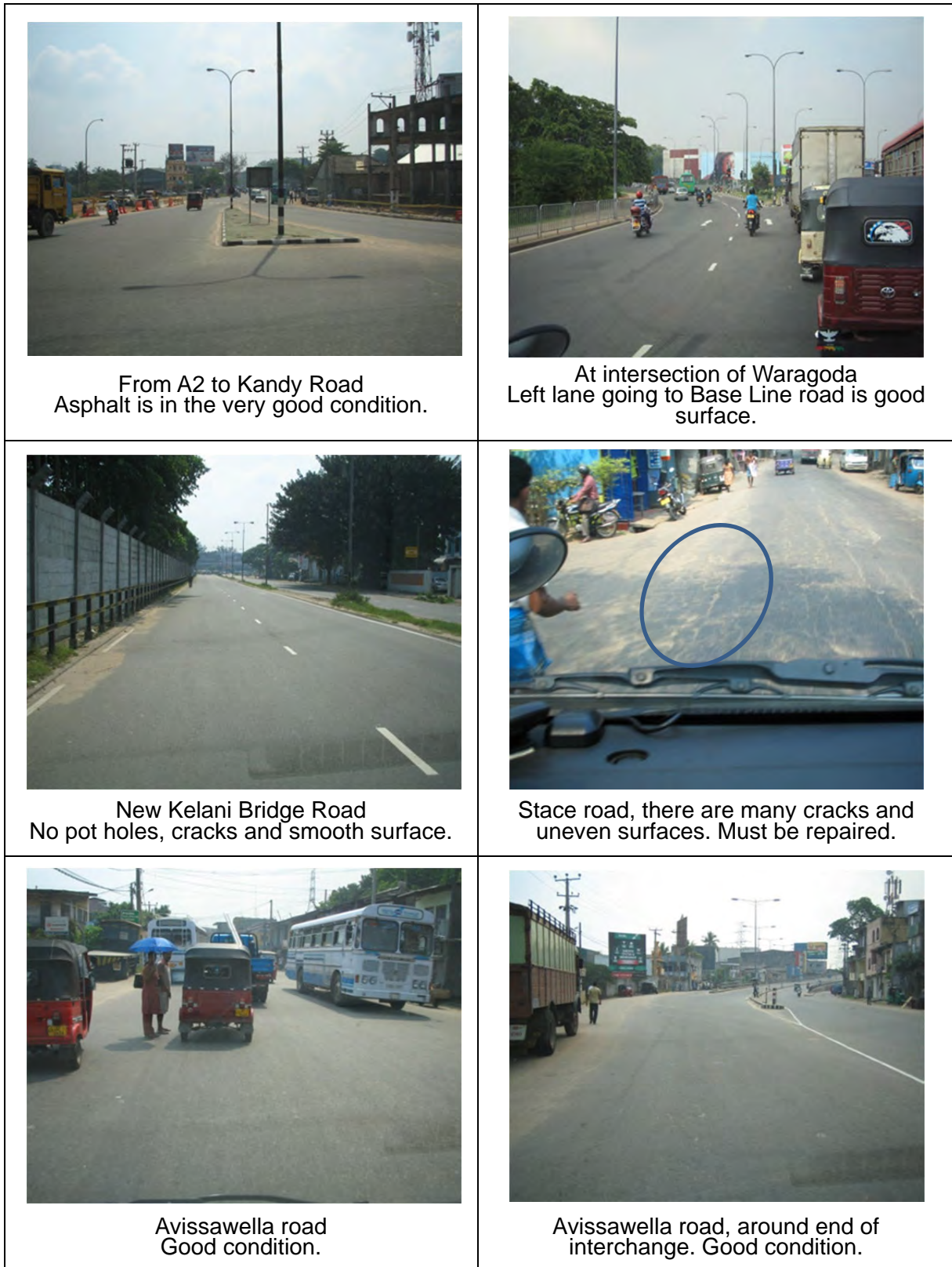
Figure 2.4.7 Extent of Damage of Road and Asphalt (2/2)
