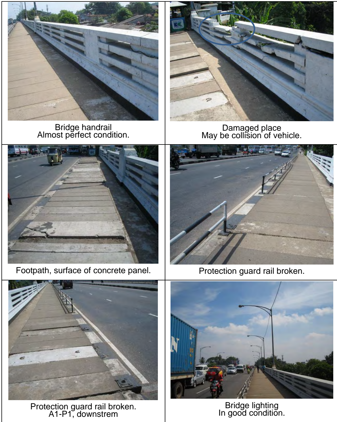
Figure 2.4.8 Other Bridge Facilities
