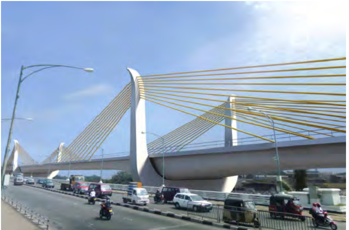
View of Main Bridge from Existing Road
