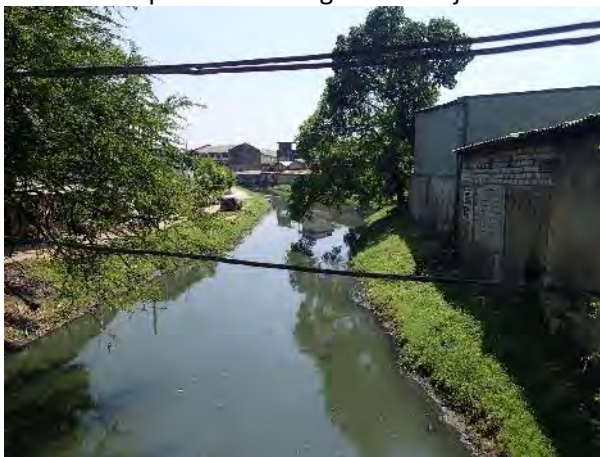
Condition of Kittampahuwa canal, near Port access road
