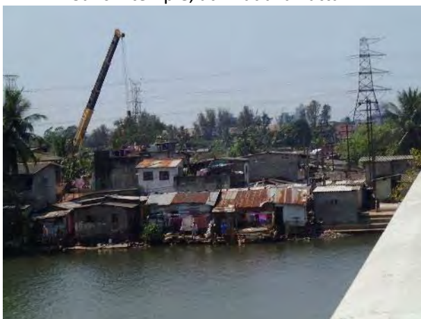
Left bank of New Kelani Bridge
