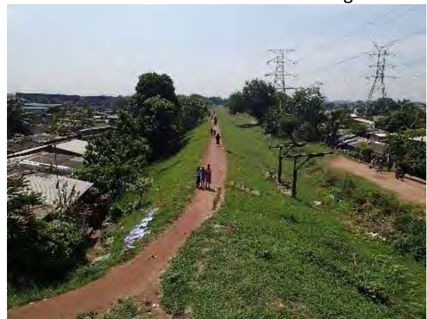
South flood bund Kelani River
