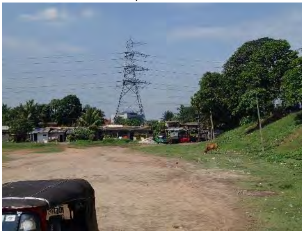
High tension power line
