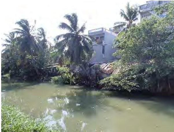
Condition of canal, near Port access road
