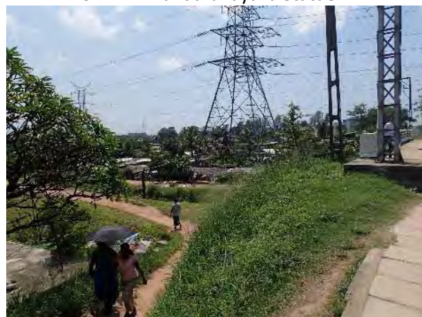
High tension power line
