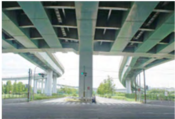
Figure 5.2.40 Some Examples of Girder Erection Completion
