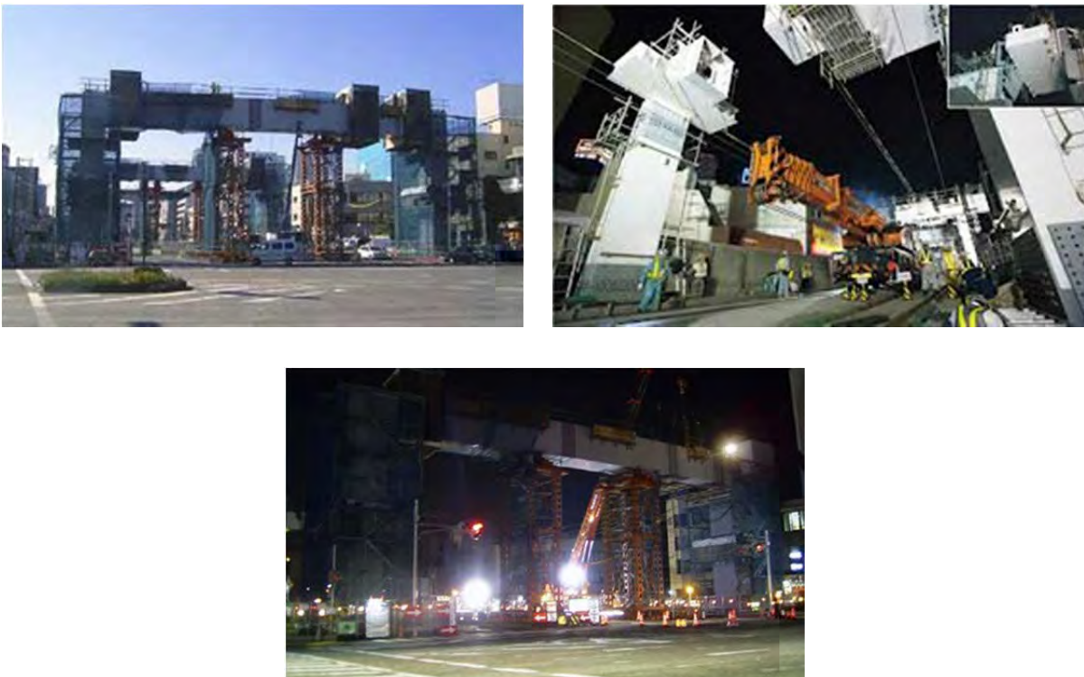
Figure 5.2.38 Some Examples of Steel Pier and Girder
