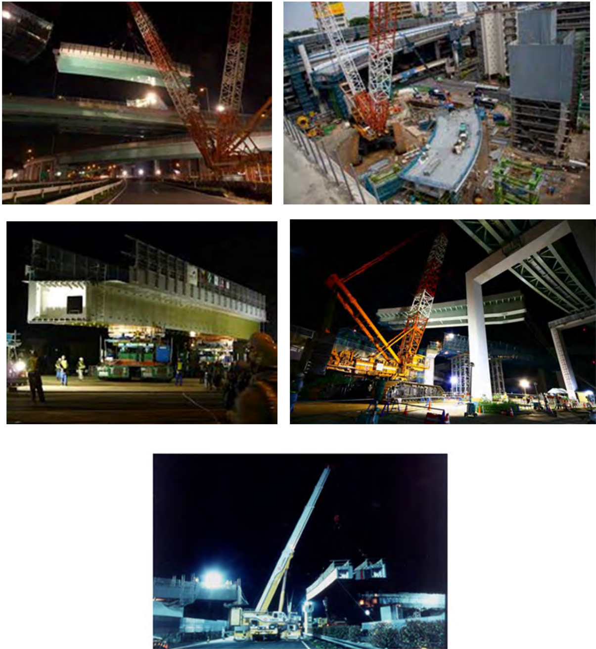
Figure 5.2.39 Some Examples of Girder Erection Work
