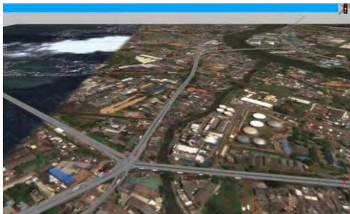
Ingurukade Interchange (Current Condition)
