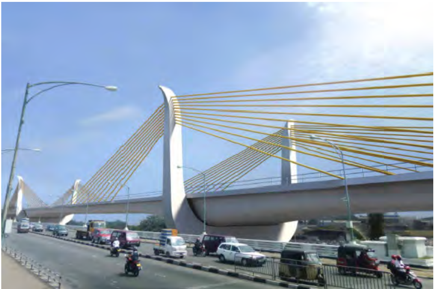
View of Main Bridge from Existing Road
