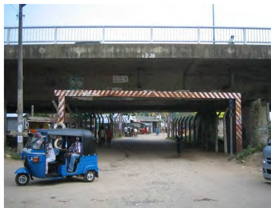
Figure 2.4.11 Example for Height Limit Guard Rail (Victoria Bridge)
