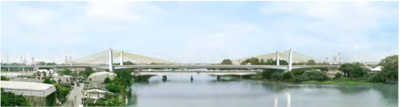
Side View of Main Bridge
