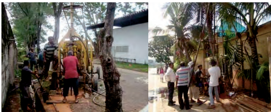
Figure 6.1.1 – Some incidents of borehole investigation
