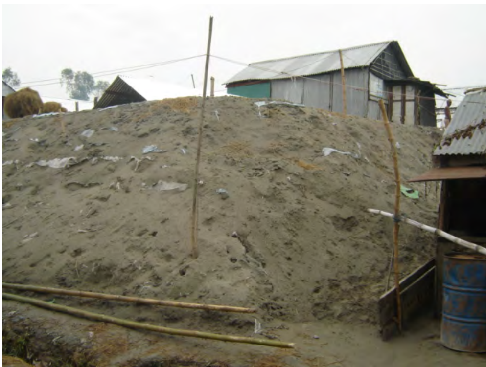
Photo 8.3 Constructed platform Side View
