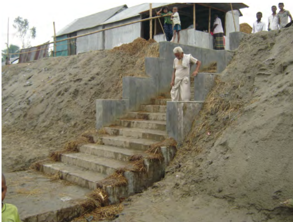
Photo 8.4 Stair to Constructed Market
