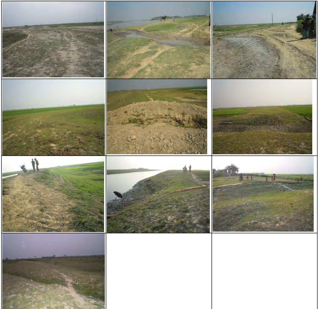
Artificial cutting and erosion due to heavy rainfall, overtop, wave action (2) Regulator
