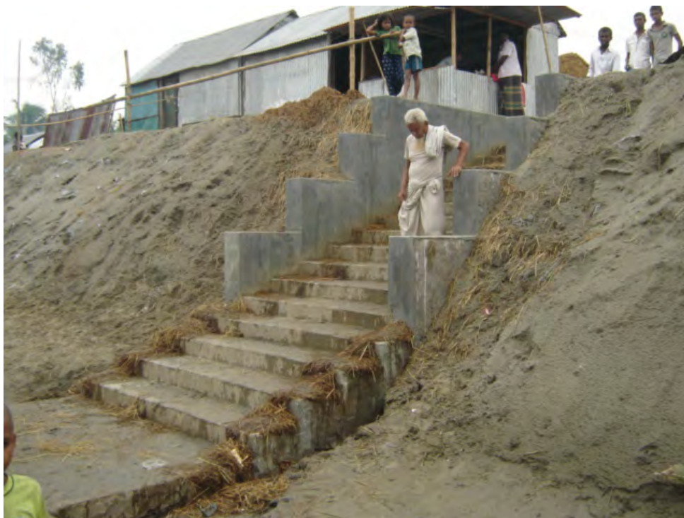
Photo 8.4 Stair to Constructed Market
