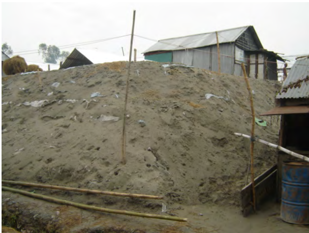
Photo 8.3 Constructed platform Side View
