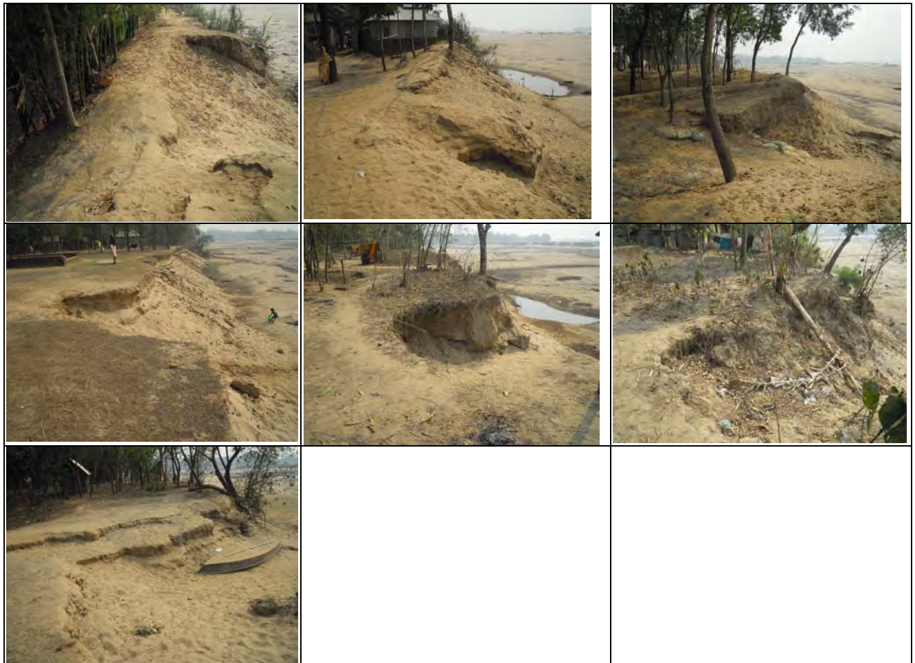
Erosion due to heavy rainfall, overtop, wave action
