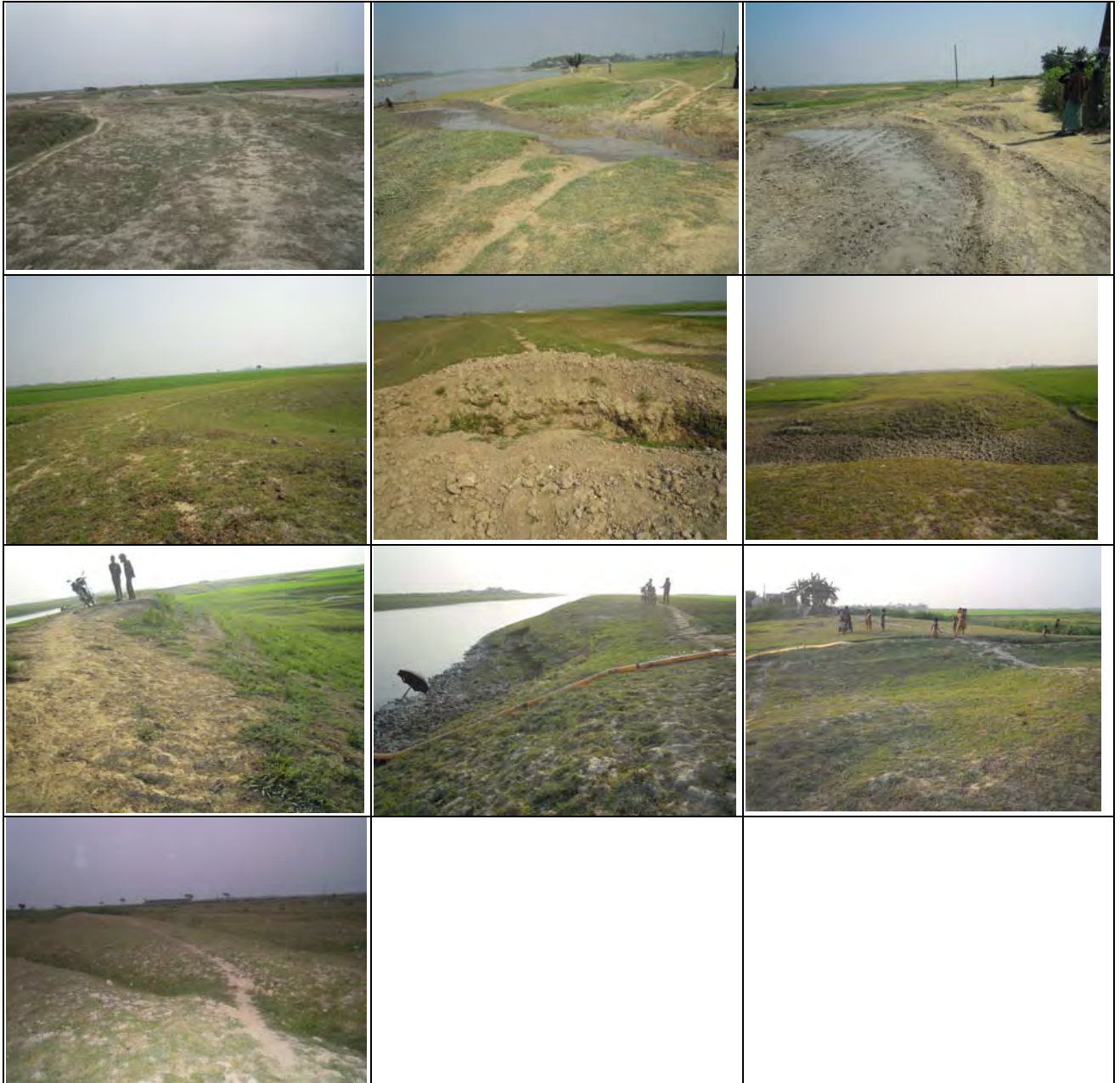
Artificial cutting and erosion due to heavy rainfall, overtop, wave action
