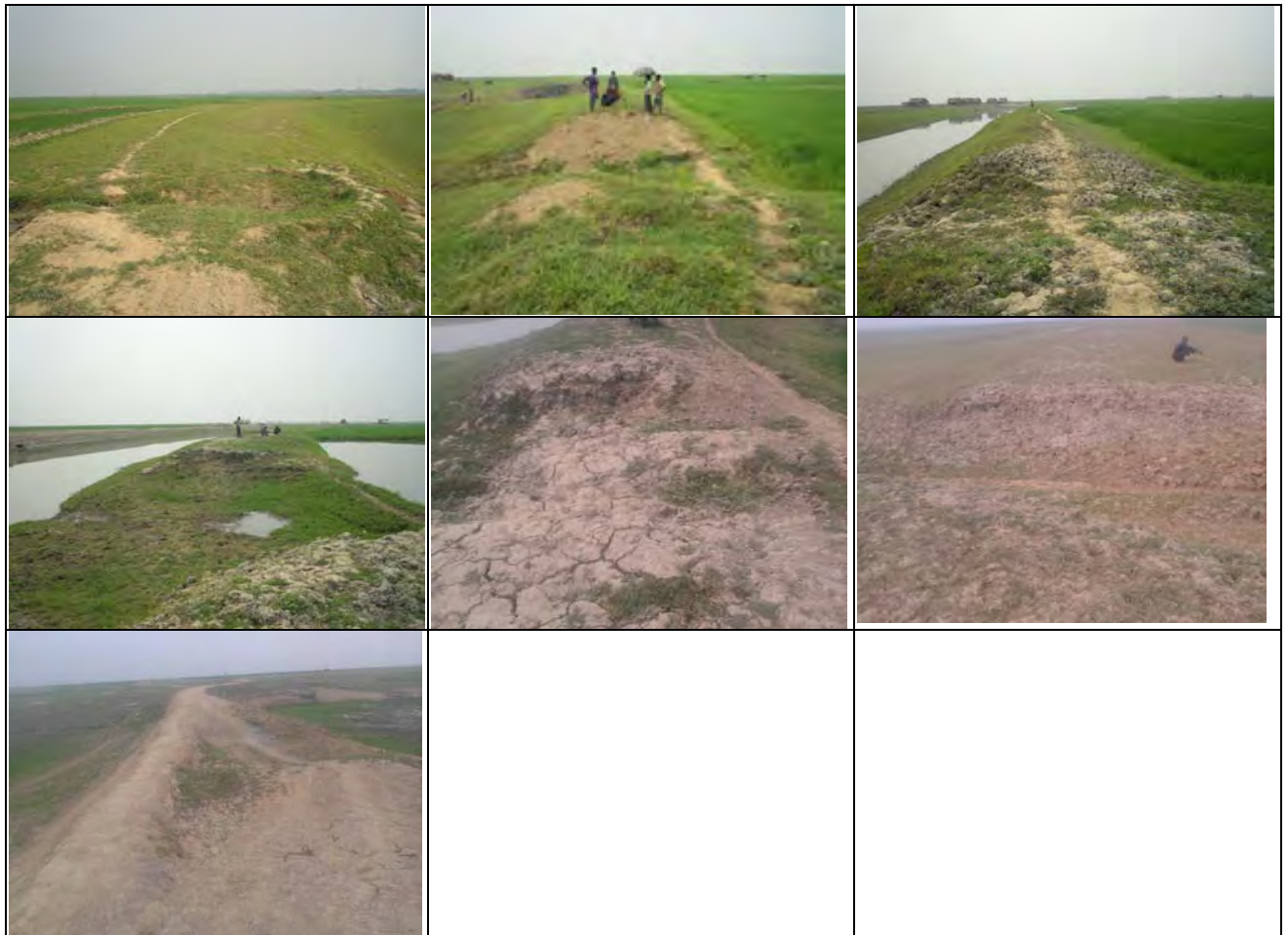
Artificial cutting and erosion due to heavy rainfall, overtop
