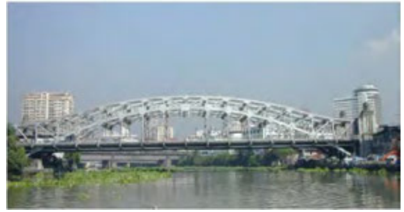
B04 Quezon Bridge
