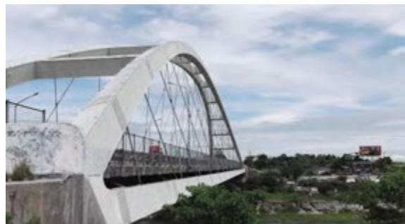
C06 Bamban Bridge
