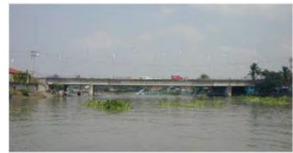
B08 Lambingan Bridge
