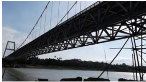
C04 Magapit Bridge
