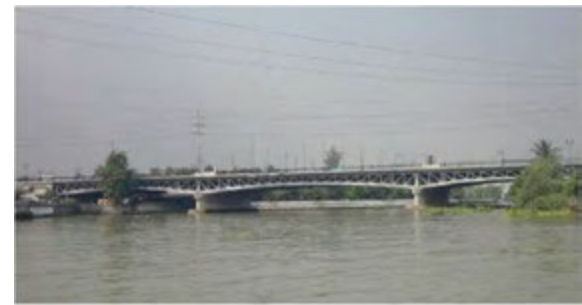
B06 Nagtahan Bridge
