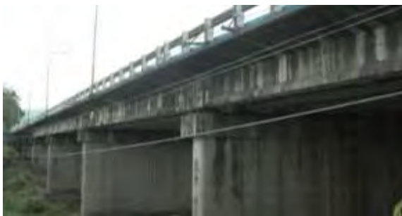
B17 San Jose Bridge
