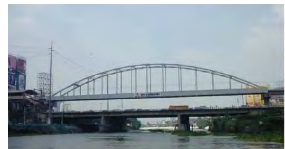
B10 Guadalupe Bridge
