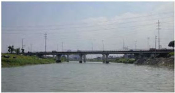
B15 Marcos Bridge
