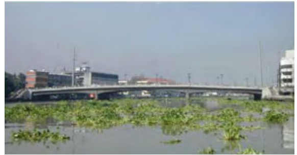
B02 Jones Bridge
