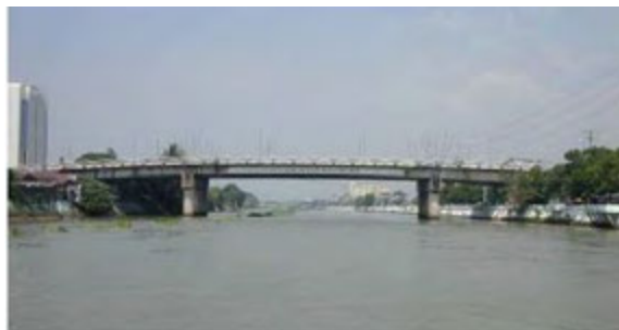
B09 Makati-Mandaluyong Bridge
