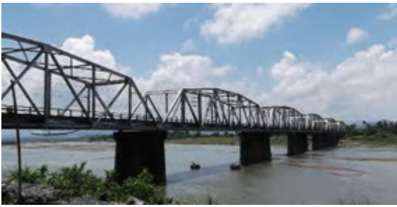
C03 Lucban Bridge
