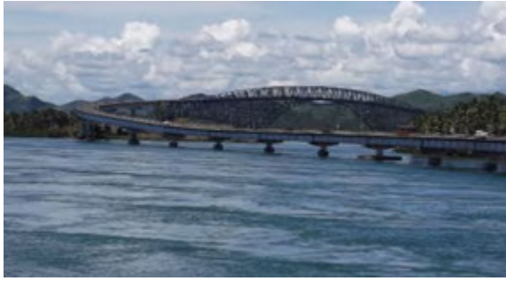
C13 San Juanico Bridge
