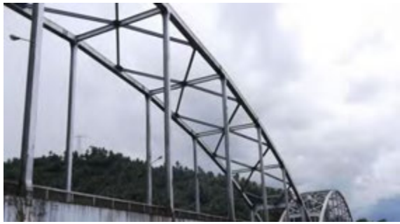
C11 Mawo Bridge
