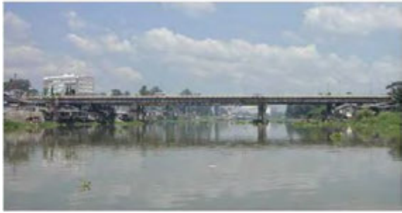
B13-1 Vargas Bridge (1 & 2)
