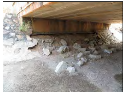
Br. 32 View on Phnom Penh Side Abutment
