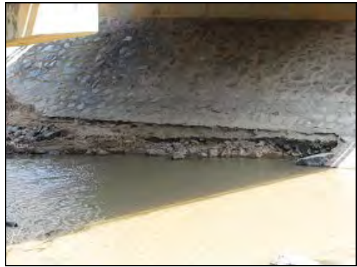
Br. 38 View on Phnom Penh Side Abutment
