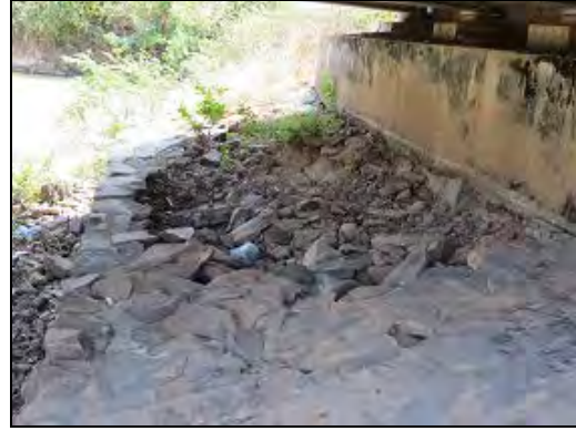
Br. 13' View on Phnom Penh Side Abutment
