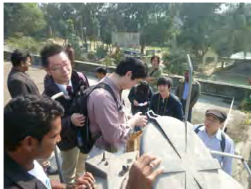
Investigation of a storage tank installed outside top of a hospital building in Manikgonji
