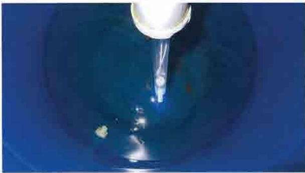
Fig5 : condition inside the tank& UV lamp
