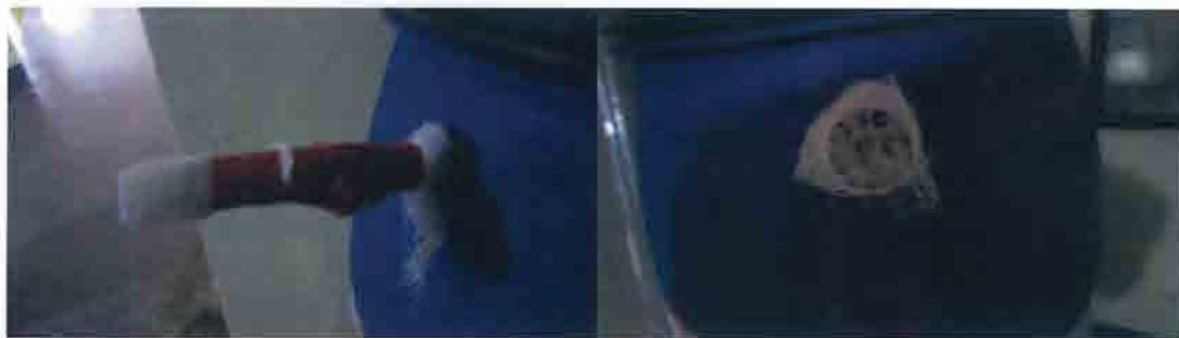
Fig 9: fixed the over flow pipe with net bag
