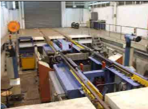
Ground Wheel Lathe
