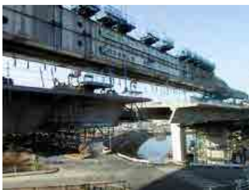
Photo 5.1-1 Construction of Girders Using Span-by-Span Method
