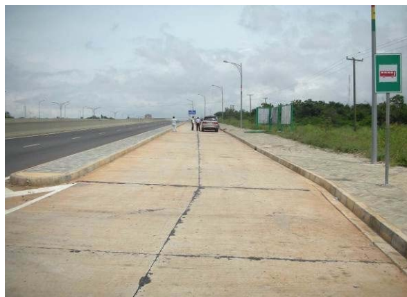
Adopted concrete pavement at Bus Bays
