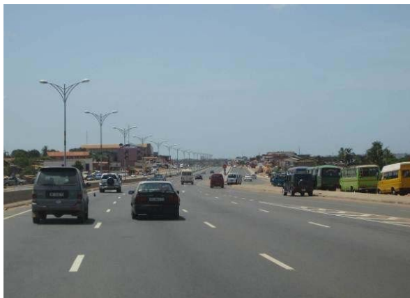
Six-lane road financed by Millennium Challenge Corporation (MCC)
