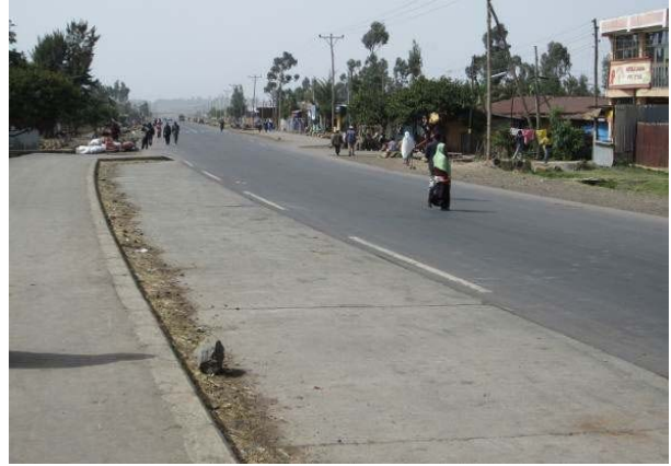
Adopted concrete pavement at Bus Bays
