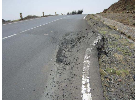
Photograph4-9. Ethiopia:Rural trunk road Pavement was failure because bearing capacity is down by influence of the groundwater from mountain side.
