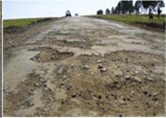
Photograph4-19. Highway section of the same area as photograph(2010 photography)
