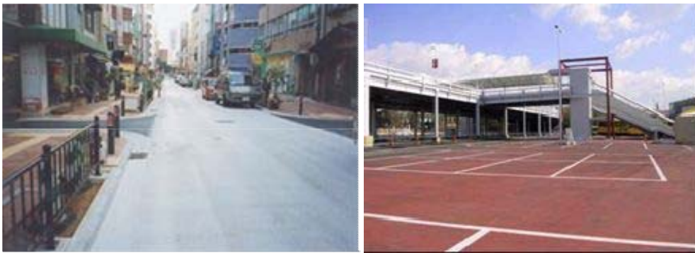
Photograph2-4. Construction example of the Semi-flexible pavement
