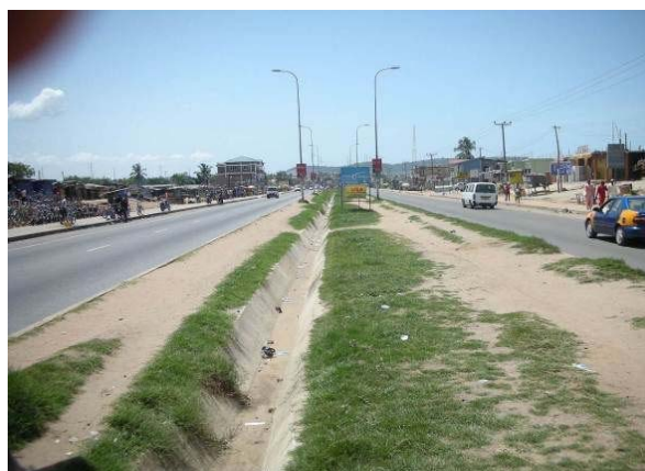
Four-lane road with wide median strip which has center drainage facilities
