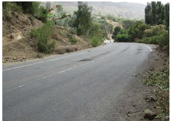
Flow rutting at sharp curve might be caused by side slip of rear tires.
