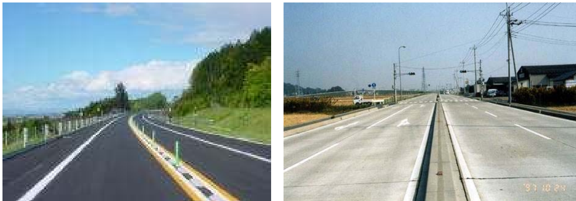
Photograph2-1 Asphalt pavement (left) and concrete pavement (right)
