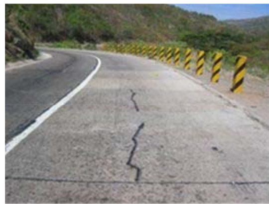
Photograph 4-25. Trunk road : Roller compacted concrete pavement(RCCP) (Tanzania)
