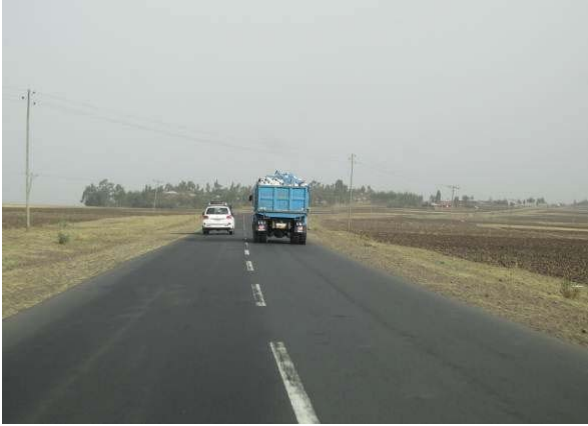
Good condition with respect to large number of heavy vehicles
