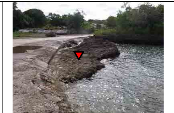
Install Area of Tide Observation System
