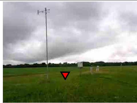
Install Area of Automatic Weather Station
