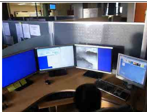
Existing terminal and display units for GTS input/output
