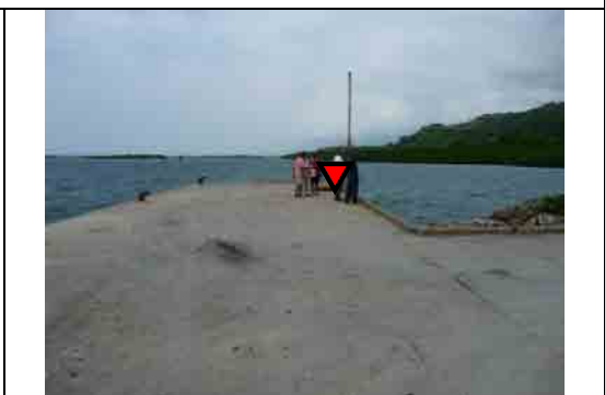
Install Area of Tide Observation System
