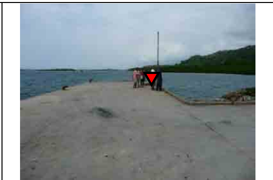
Install Area of Tide Observation System
