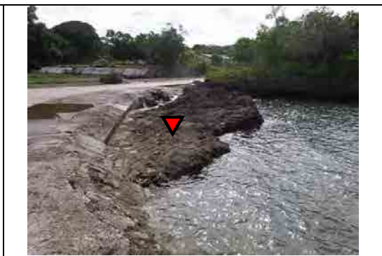
Install Area of Tide Observation System
