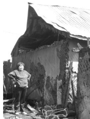
Figure 5.5.25 View of house 2 from Ger
