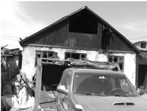
Figure 5.5.24 Southside view of house 2
