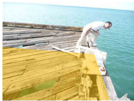
Install Area of Tide Observation System
