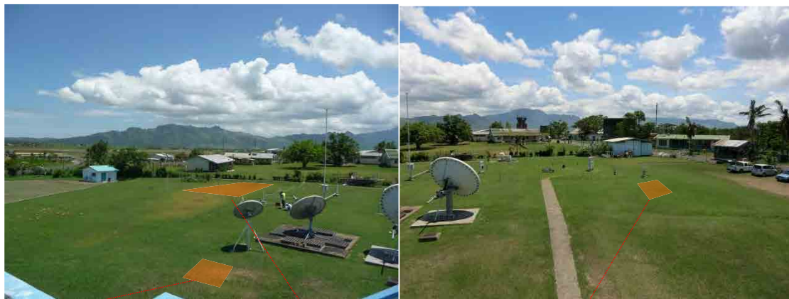
VSAT Communication System
