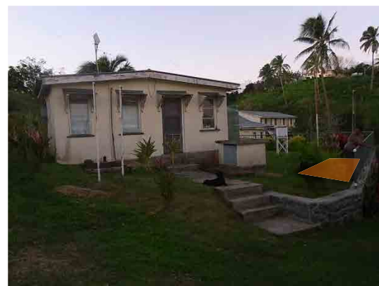
Install Area of Lightning Detection System
