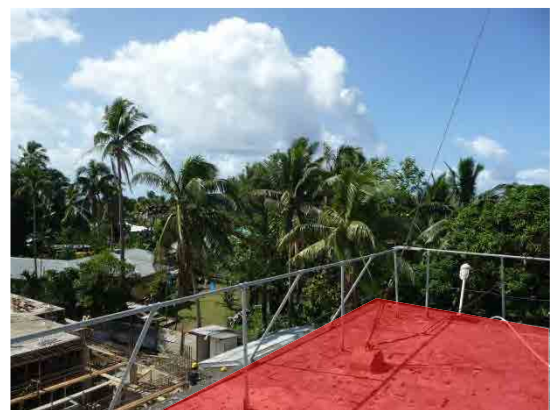
Install Area of Lightning Detection System
