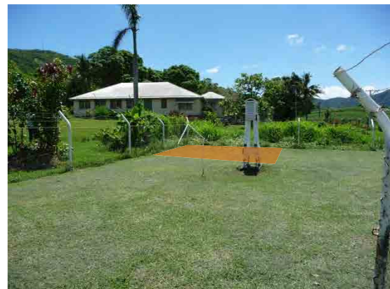
Install Area of Lightning Detection System
