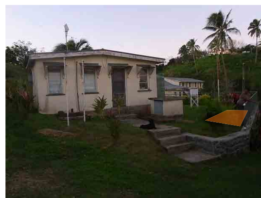
Install Area of Lightning Detection System
