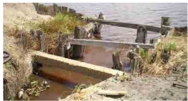
PH2-1-17 Revetment at the inlet mouth
