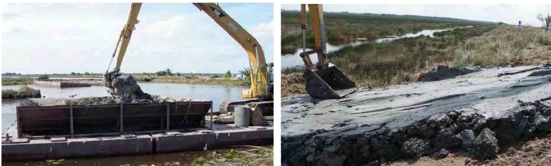
Ph.10-1 In-situ mixing test of Soil cement at the Preparatory study
