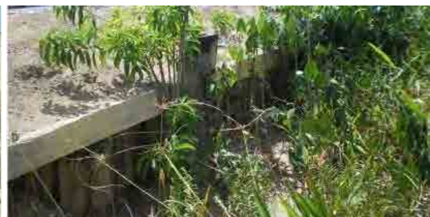
PH2-1-19 Revetment at the outlet mouth
