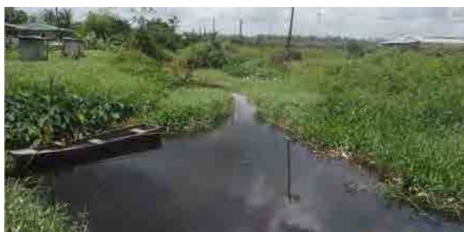
PH2-1-26 Canal condition at the downstream of the regulation gate
