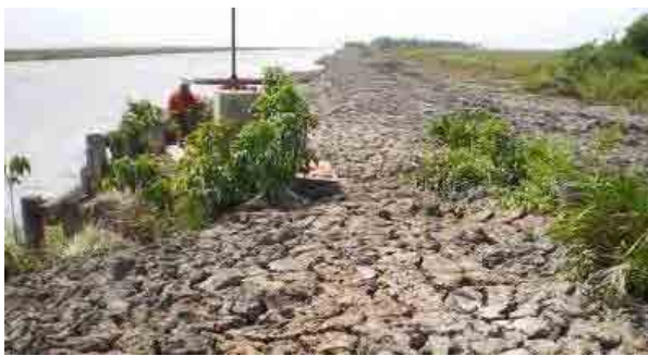
PH 2-1-5 Embankment crest and the spindle
