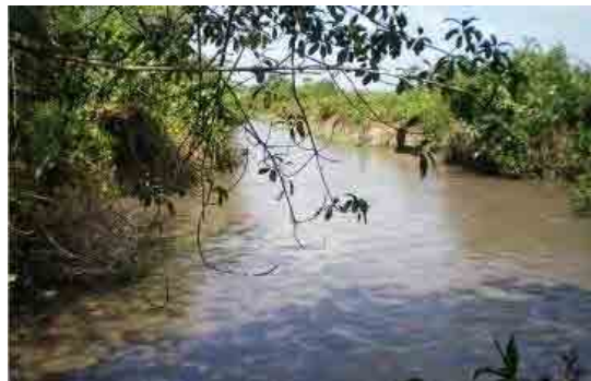
PH 2-1-3 Canal flow maintained by leakage water
