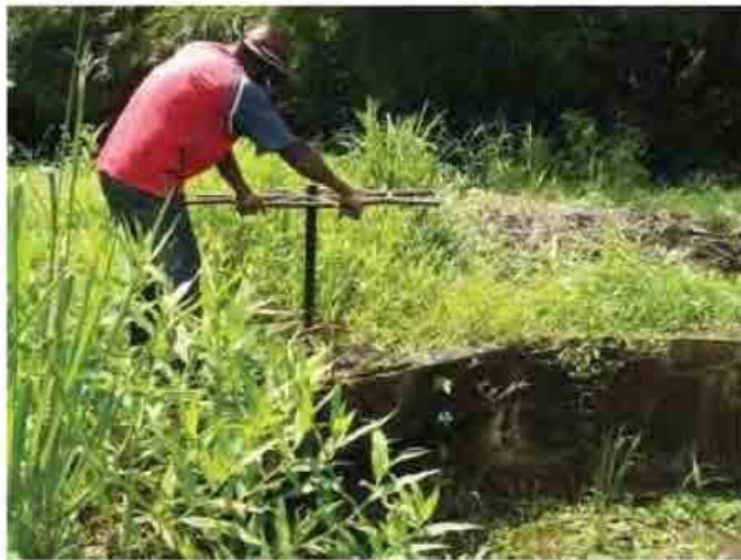
PH2-1-14 Gate operation and the retaining walls
