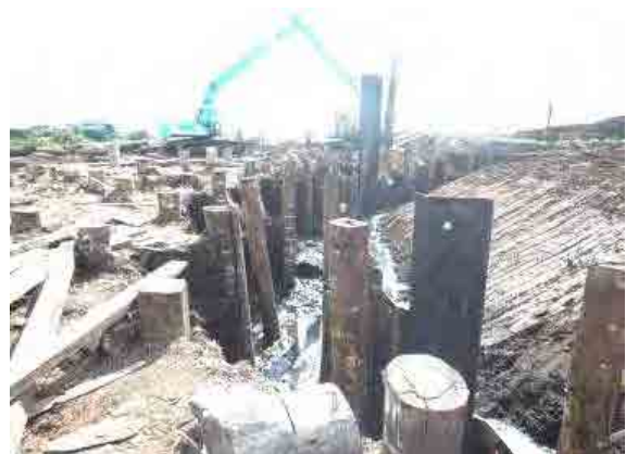
PH2-1-36 Pile driving works as the foundation treatment for the sluice structure at the beginning of the canal
