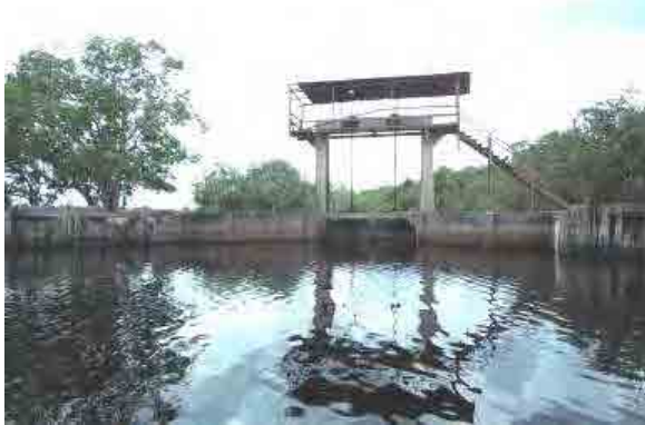
PH2-1-27 Gate and the retaining walls
