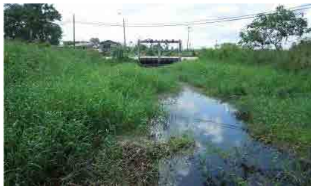
PH2-1-23 Canal condition at the upstream of the Johanna regulation gate
