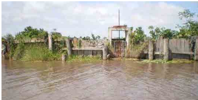
PH 2-1-7 Wooden pile revetment at the upstream side
