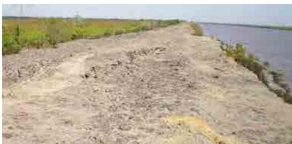
PH2-1-20 Steps caused by sliding
