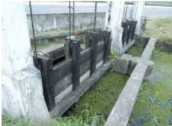
PH2-1-22 Culvert channels, gates and winch systems
