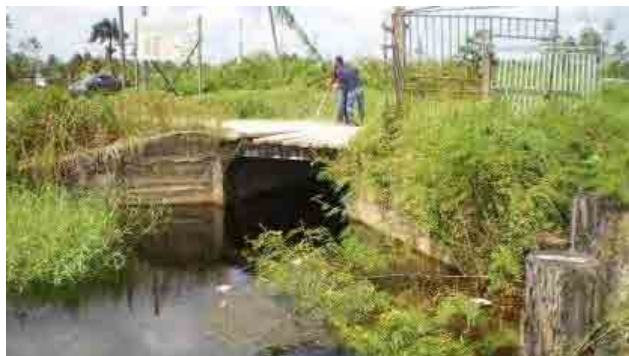
PH2-1-25 Wooden bridge and the narrow concrete flume
