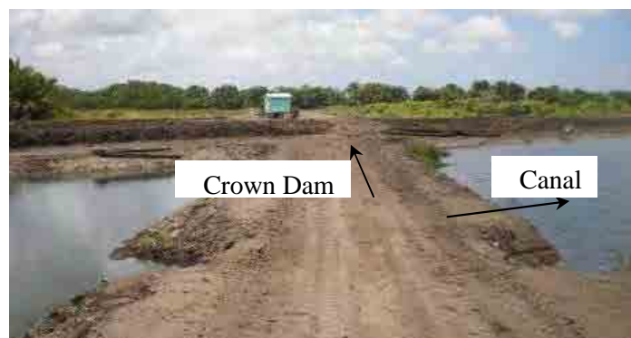
PH 2-1-38 Crossing point of the Crown Dam and the Hope/Dochfour canal
