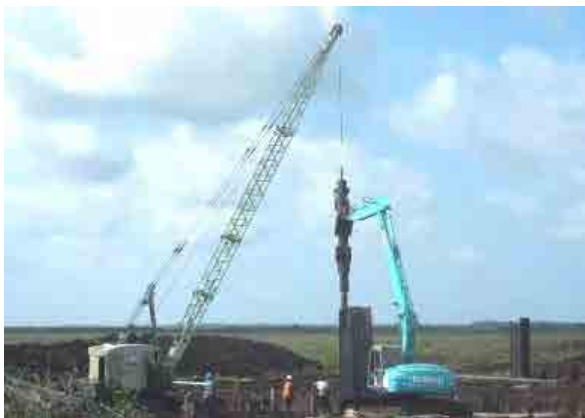
PH2-1-36 Pile driving works as the foundation treatment for the sluice structure at the beginning of the canal
