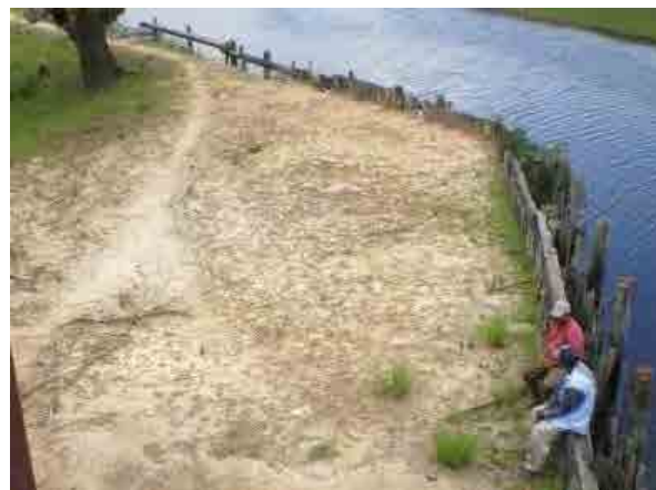
PH2-1-31 Embankment surface composed of well-compacted clayey soil
