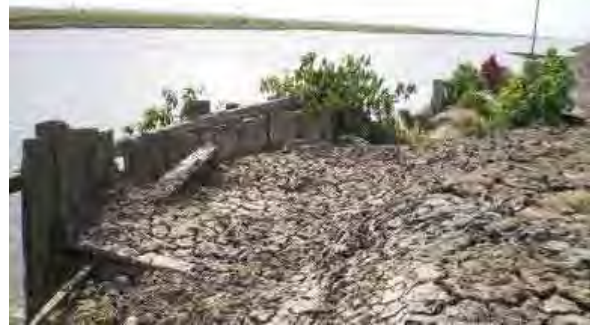
PH2-1-6 Wooden pile revetment at the inlet mouth
