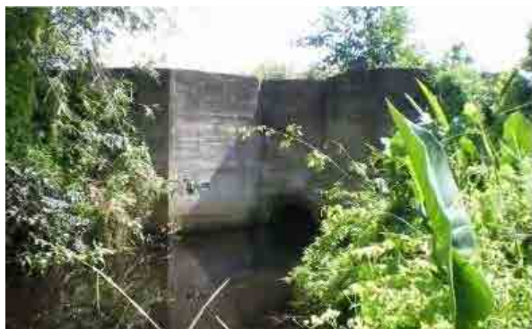
PH2-1-12 Retaining walls at the outlet
