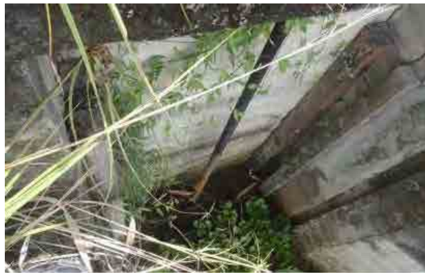
PH2-1-10 Spindle attached to the gate
