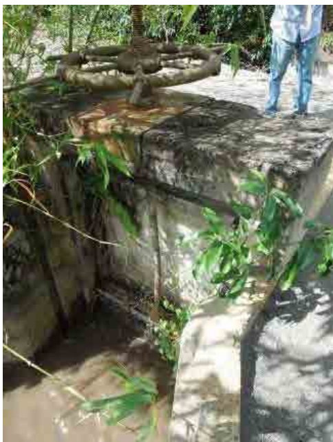
PH 2-1-1 Bent of the spindle
