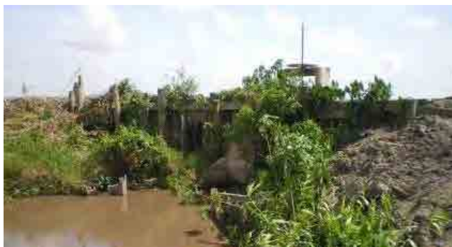
PH 2-1-8 Wooden pile revetment
