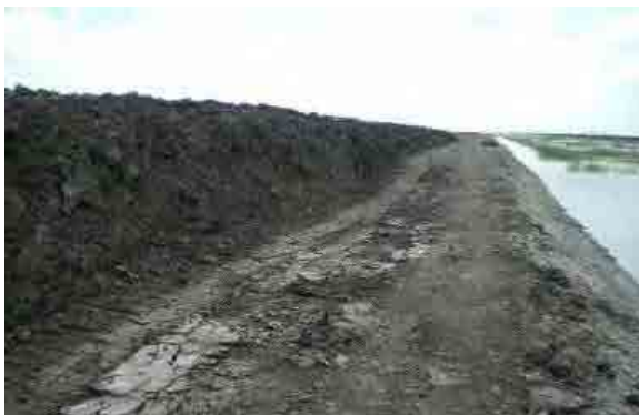
PH2-1-35 Canal excavation and the stockpile of the embankment materials at the point about 2 km from the conservancy
