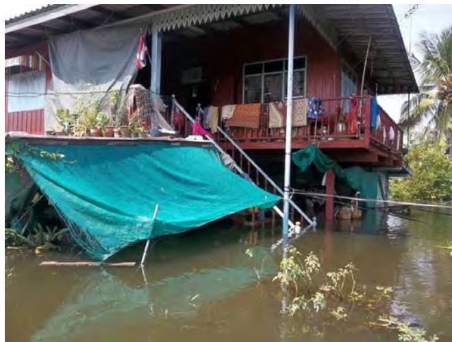
Figure17Flooding around housing area
