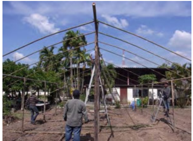
Main structure is almost done. (Dec. 23, 2012)
