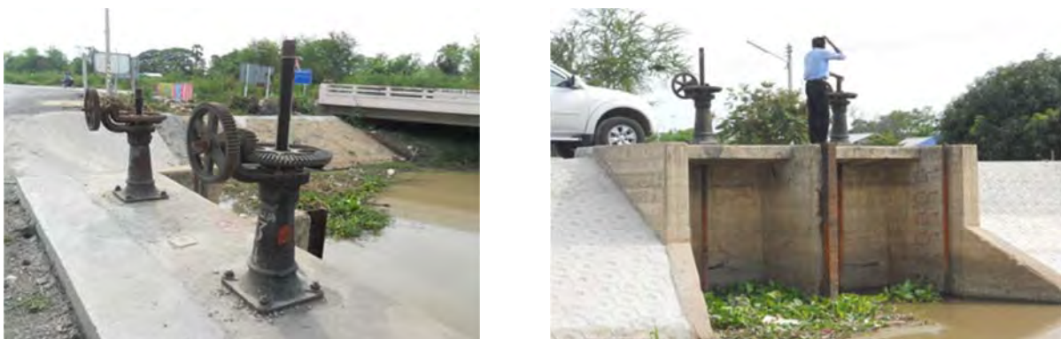
Fig: The Water Gate of the 5th Collector Drain
