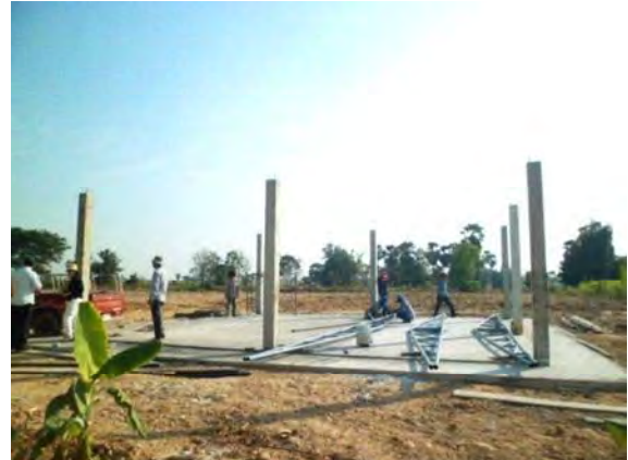
Installation of Columns
