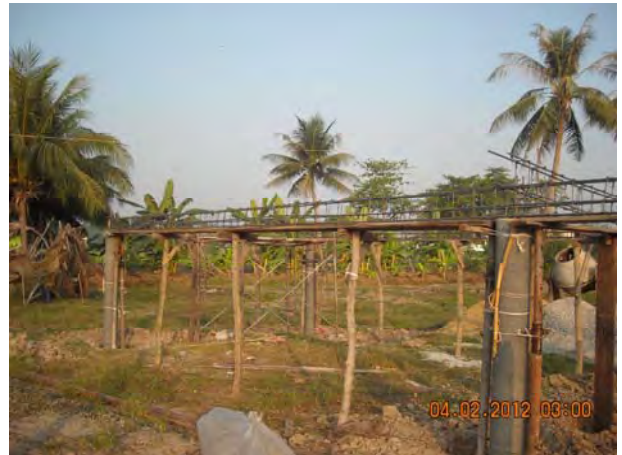
Goat House under Construction
