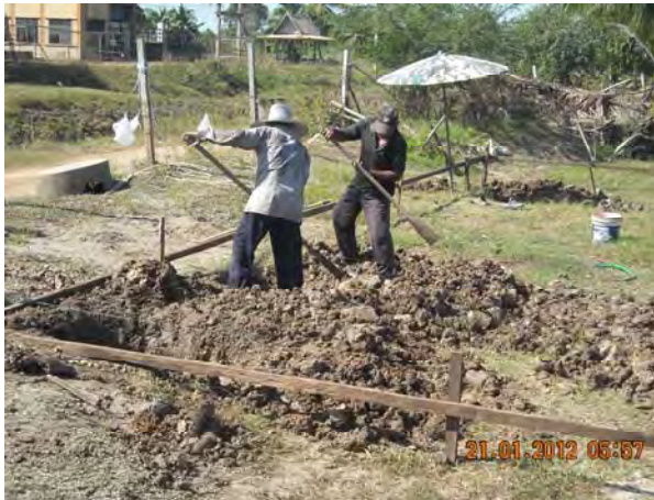
Commencement of the Work
