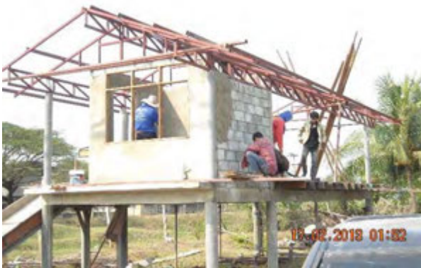
Goat House under Construction
