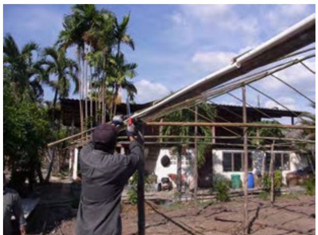
Plastic pipes were set to fix the saran net. (Dec. 23, 2012)
