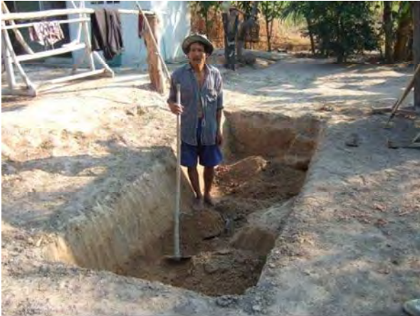
Excavation of the Pit by a Beneficiary
