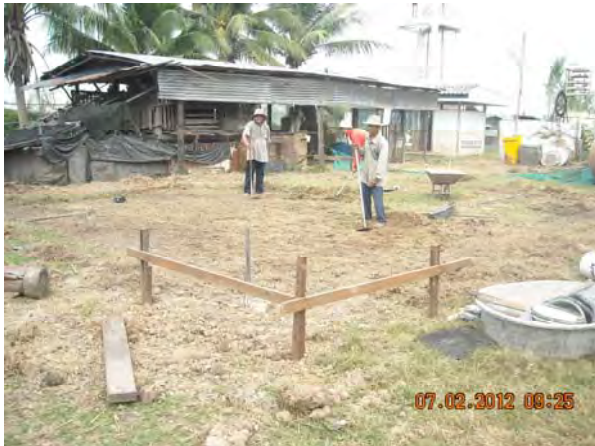
Commencement of the construction
