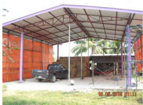
Completed Feed Storage
