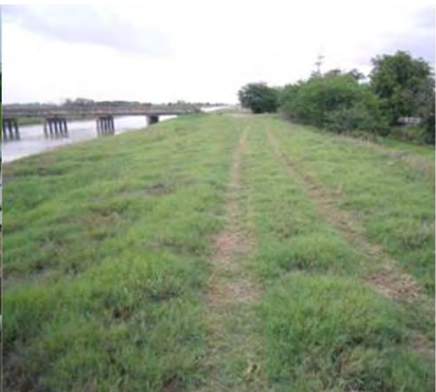
Dike along Water Supply Canal
