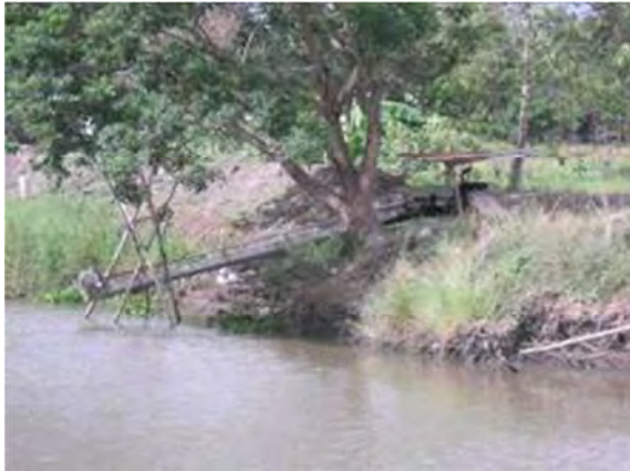
Pumps used for pumping water into fields
