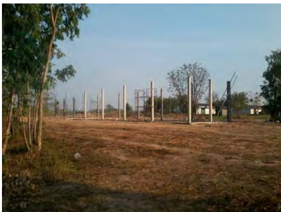
Silage storage under construction
