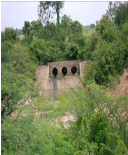
Changing the drain tubes of MC Canal to improve the flow.
