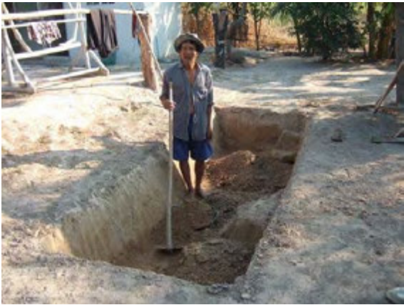
Biogas under installation
