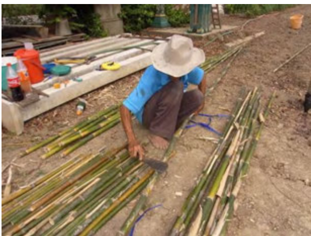
For safety reason, surface of the bamboos was smoothed. (Jan. 30, 2013)
