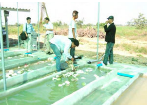
Monitoring the construction
