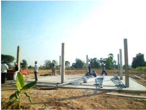
Feed storage under construction
