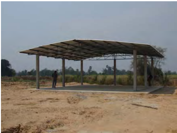
Completed feed storage
