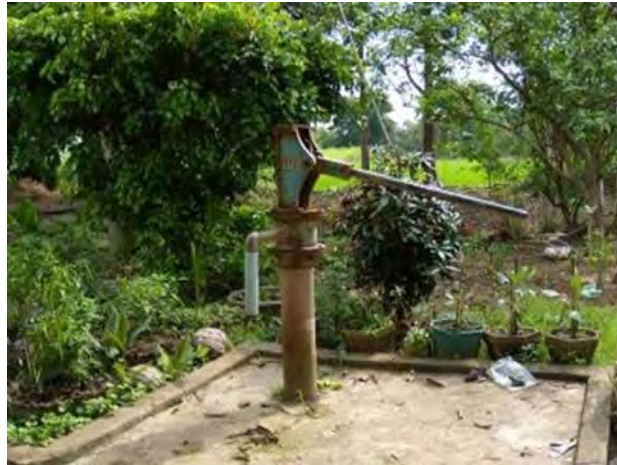
Figure 7 Artesian Well/ Hand Pump
