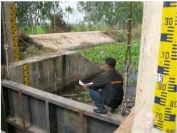
Installed staff gage
