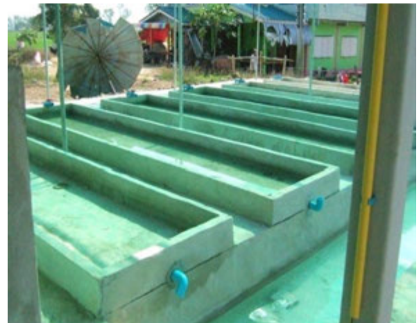
Aquaponics System (During Construction) 2
