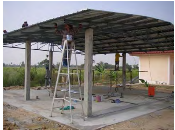
Feed storage under construction
