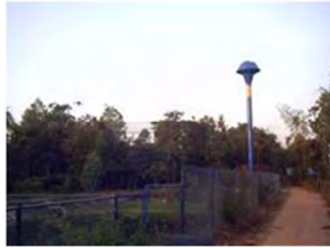
Fig: Water tank
