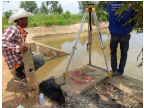
Benchmark survey by contractor
