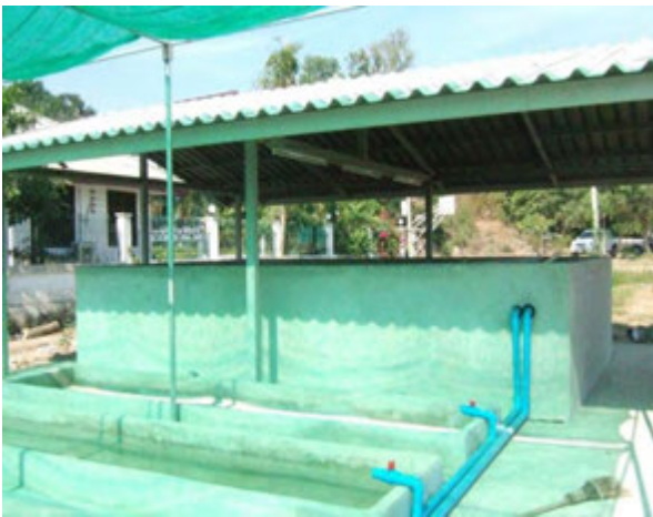
Aquaponics System (During Construction) 1
