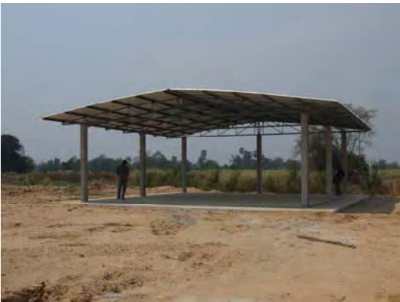
Completed feed storage
