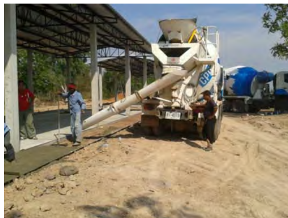
Silage storage under construction
