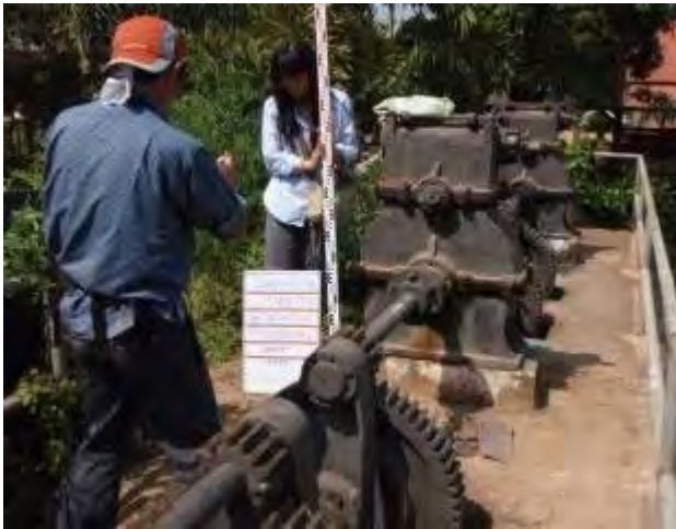
Gate and gear inspection
