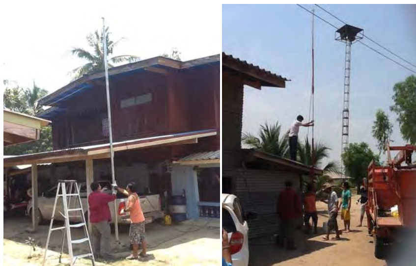
Installation of the signal station at 12 locations
