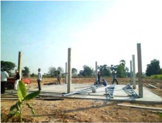
Feed storage under construction
