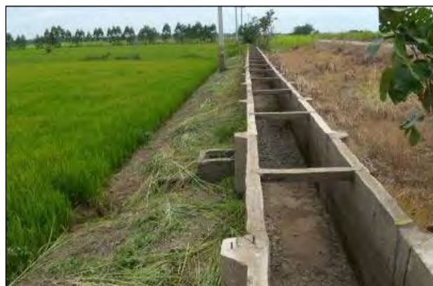
Electric Pumping and Distribution System of Moo 9 is built a sink out taking water to a concrete canal so called Klong Dard
