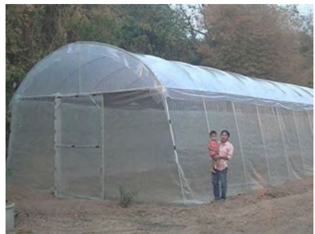
Outward appearance of the Type-A net house; it can prevent insects, mitigate strong sunshine, and avert excessive rainwater during rainy season. (Jan. 24, 2013)
