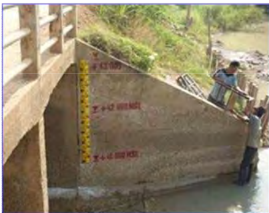
Staff gage installation work
