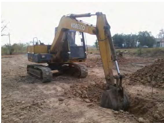
Civil work (excavating)
