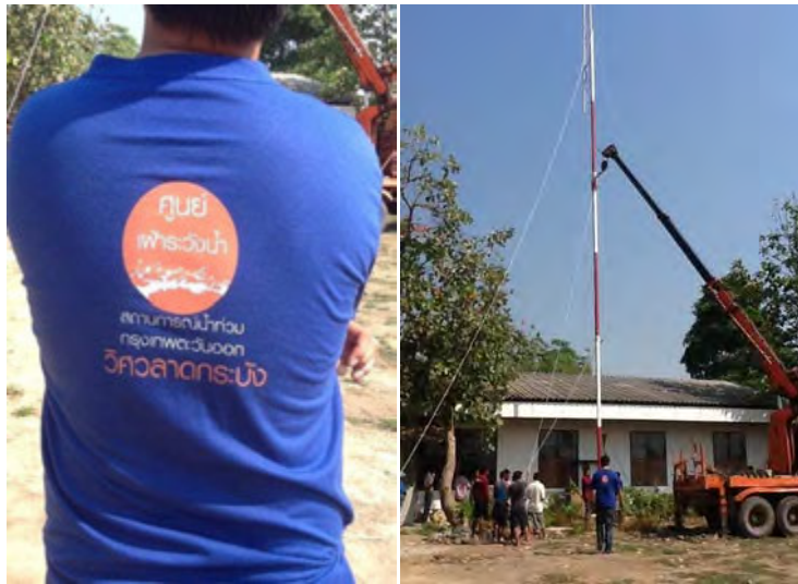
Ladkrabang Engineering Disaster Surveillance Team supported on the communication system installation
