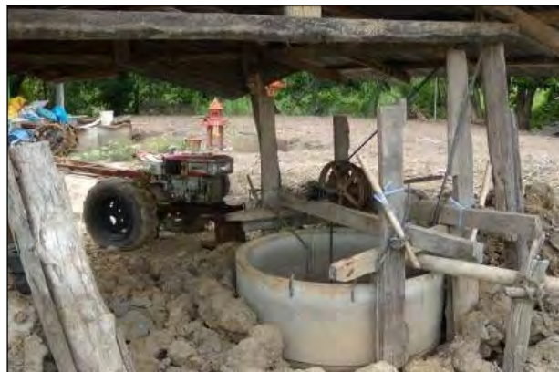
3 Electricity Pumping Projects in Village Moo 9 Ban Taback Ngam
