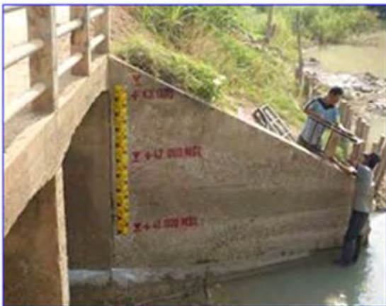
Staff gage installation work
