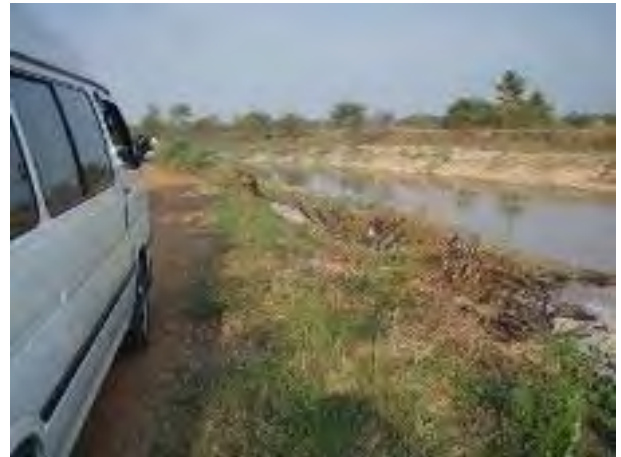
Drainage canal 6ht February 2013
