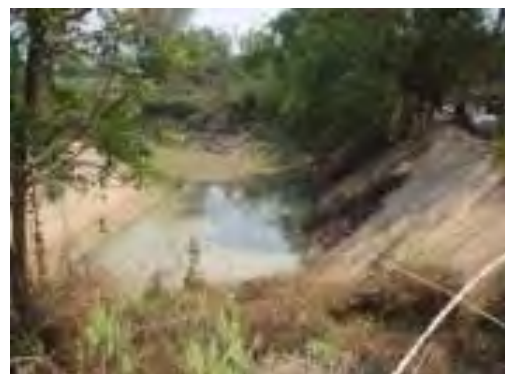
Intake facility constructed by SSIP in Muban 5 in Wang Man Canal A part of slope protection was collapsed.
