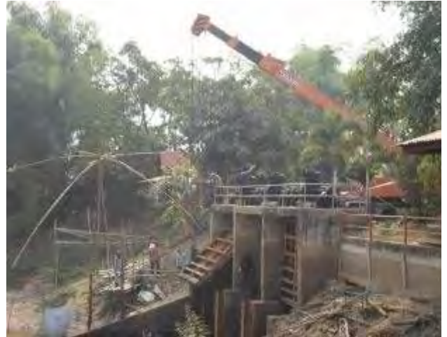
Commencement of gate repair work by RID and TAO
