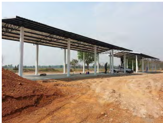
Silage storage 100% completed
