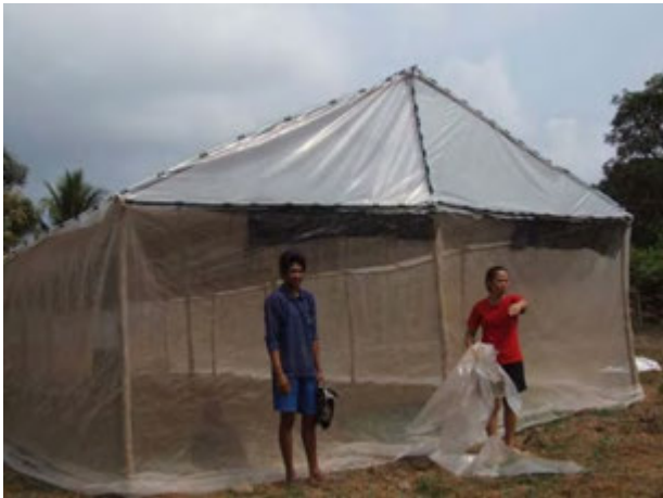
Another type of net house, called Type-B was constructed; main structure of which is made of what is locally available with cheap price. (Jan. 24, 2012)
