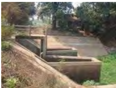
Intake facility constructed by SSIP in Muban 5 in Wang Man Canal A part of slope protection was collapsed.
