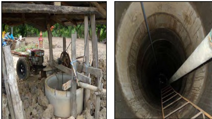
Figure 5 Artesian Wells in Chum Saeng Songkhram Sub-district
