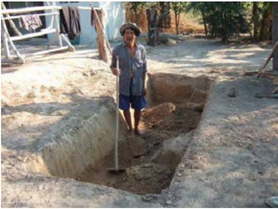
Biogas under installation
