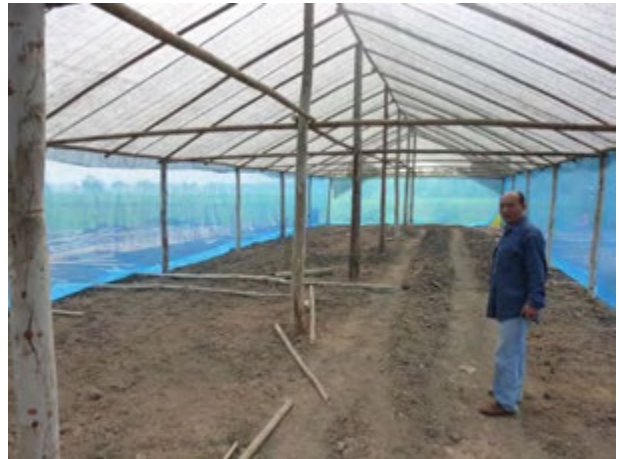
Type-C is made of saran net for roofing. This particular one has a surrounding walls made of plastic net for insect prevention. (Jan. 24, 2013)
