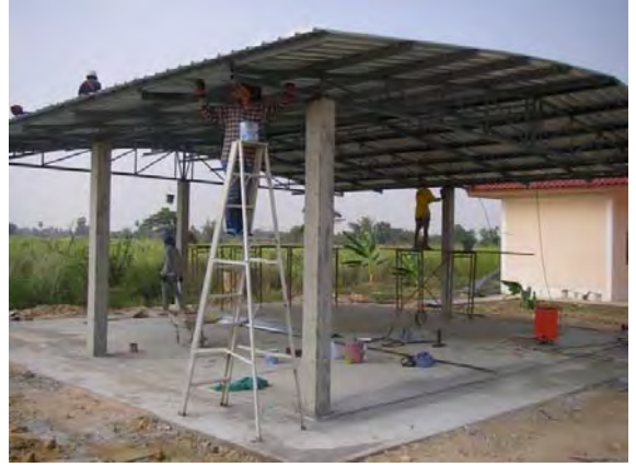
Feed storage under construction
