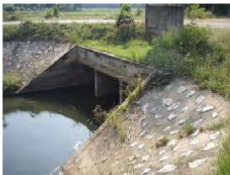
Small Scale Irrigation Project Wang Man Pipe Regulator Mar 7 th 2013 Weed ridden canal and not well maintained
