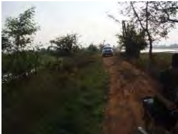
Site of repairing dyke, 6ht February 2013
