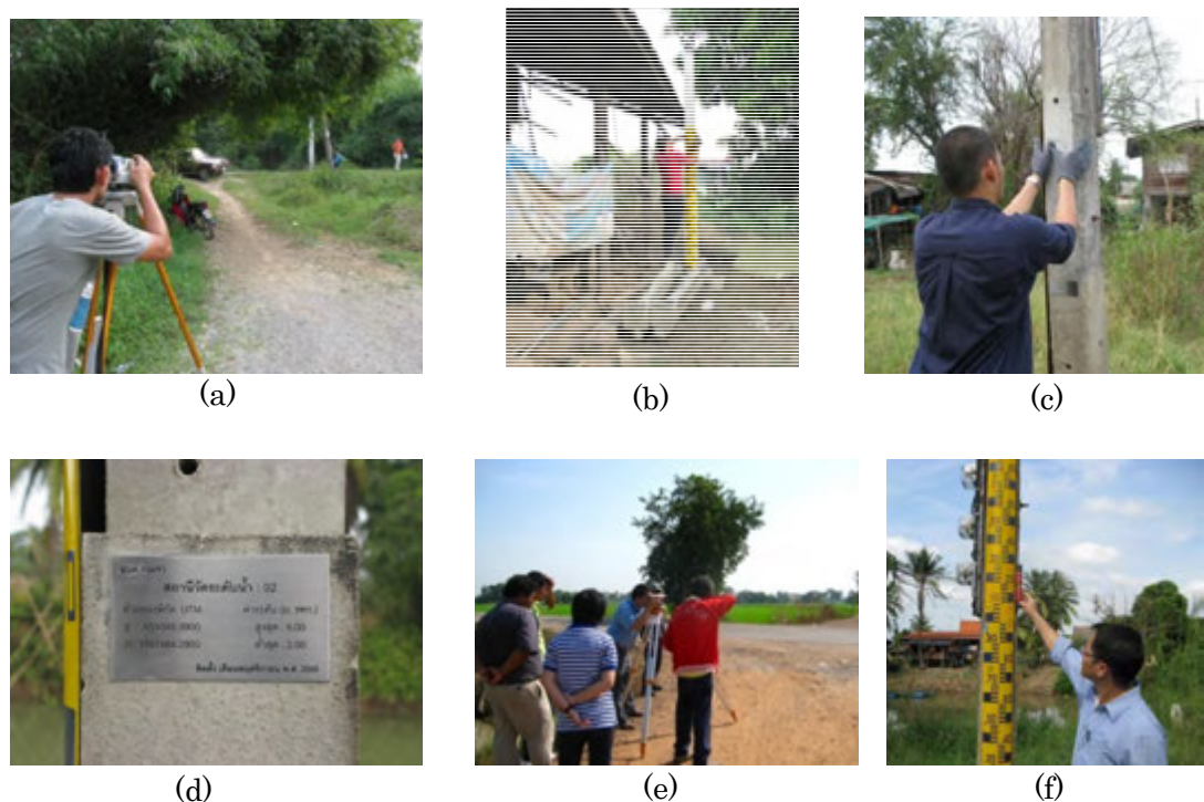
Figure 5. Examples of the staff gage installation process (a) transfer the reference ground elevation to the staff gage station, (b) staff gage installation, (c) installation of staff gage station tag (d) an example of a staff gage station tag (e) inspection of staff gage elevation and (f) final inspection of workmanship
