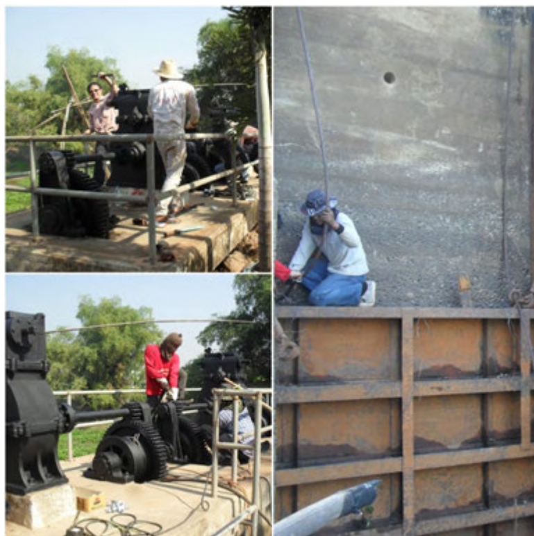
4. A new steel sling was installed in order to lift up the 3 gates to be repaired.
