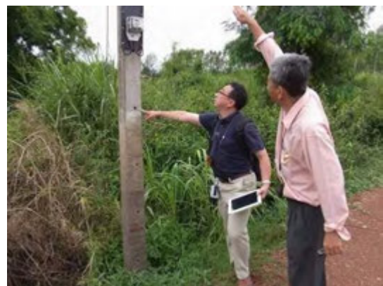
Due to highly elevated water level, electricity meters needed to be replaced at way higher place, which may not be easy to read.
