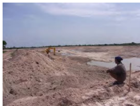
A new farm pond being excavated at a middle part of the Tambon; in upland places, securing water is a crucial issue.
