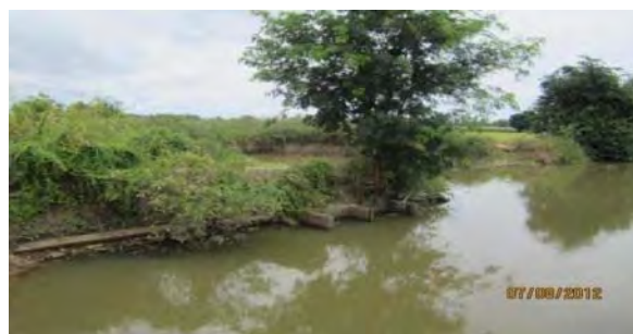
2012/8/7, Head regulator for the right main canal
