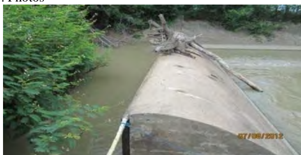
2012/8/7, Nong Kai Lai Weir
