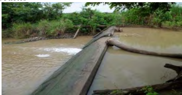
2012/7/28, Khlung Nam Lat Weir
