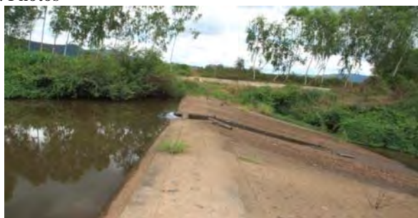
2012/6/29, Nam Phak Noi Weir and outlet
