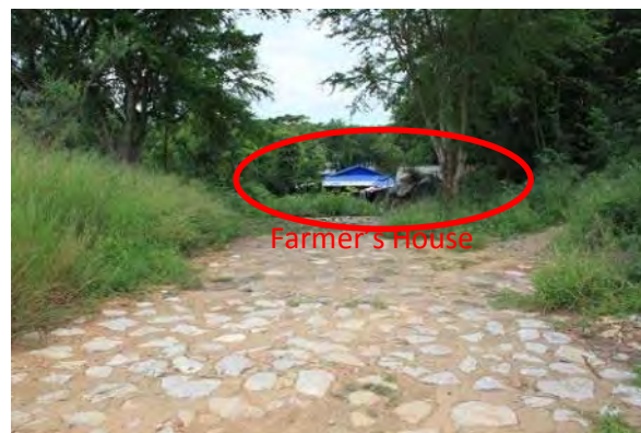
2012/08/01, Spillway of Kham Ta Khian Reservoir
