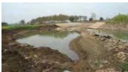
No69 Downstream of the weir
