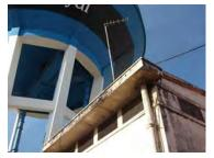
b. UHF antenna on substation
