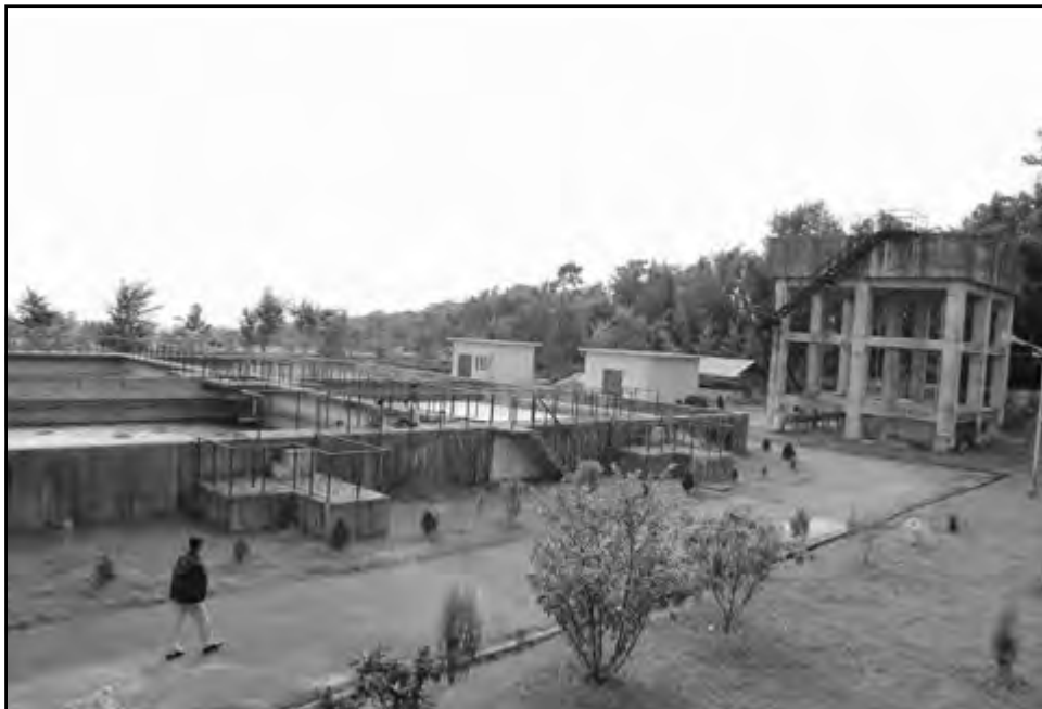
Water treatment plant and No.1 elevated tank
