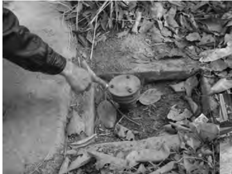
Air valve chamber without cover
