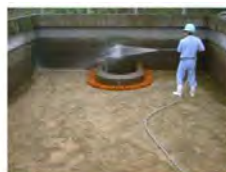
2. Clearing of walls Removing dirt on the walls
