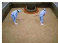
5. Preparing the surface evenly
