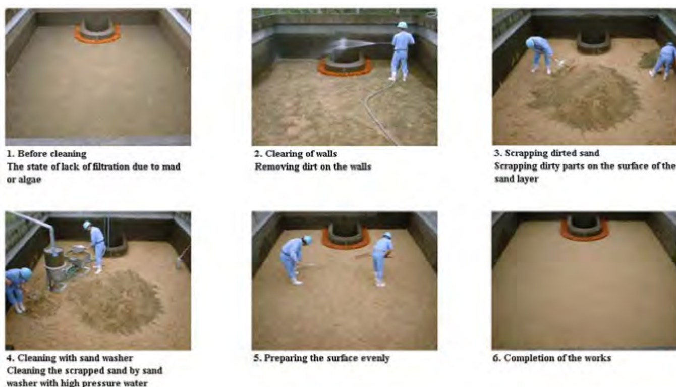
Figure-8: Example of Sand Scraping Works in Japan
