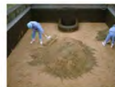
3. Scrapping dirtied sand Scrapping dirty parts on the surface of the sand layer
