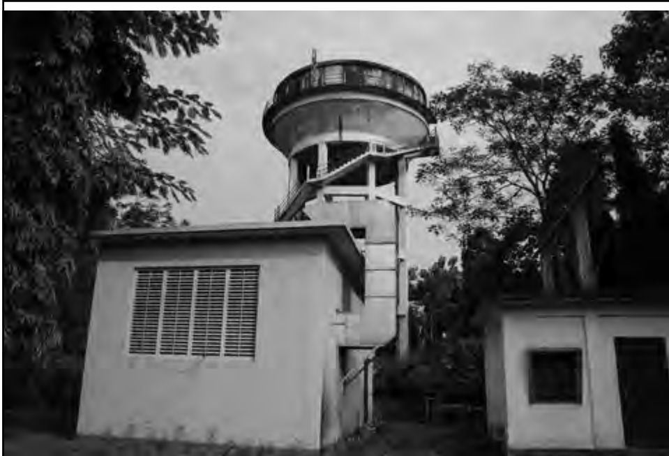
No. 2 elevated tank
