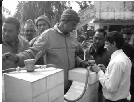
Checking if any leakage at the connection points
