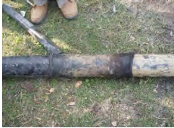
Installation of socket completed.
