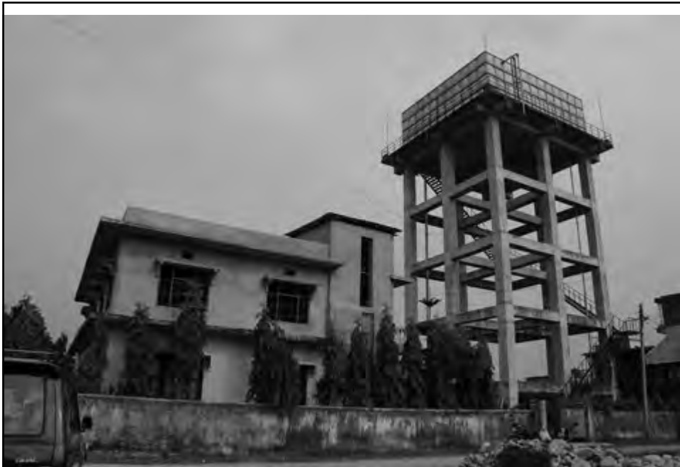
NO. 3 Elevated tank and WUSC office Building
