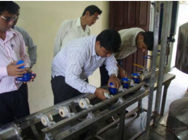
Setting WUSCs' water meters in the calibration equipment
