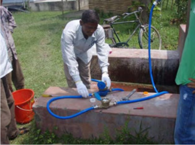
Connecting the water meters
