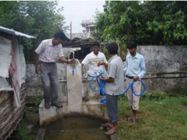
Connecting the water meters
