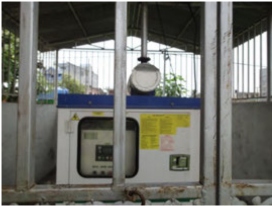
(13) Newly Installed Generator (Itahari)
