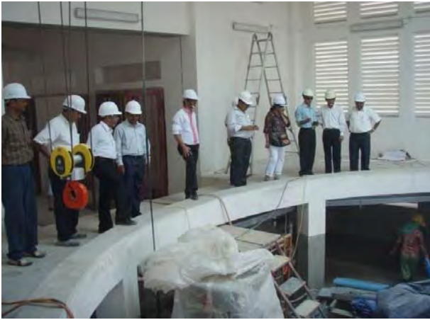
Photo-6 Third country Training in PPWSA in Cambodia Water Treatment Plant construction site visiting Installation of pumps in the intake facility
