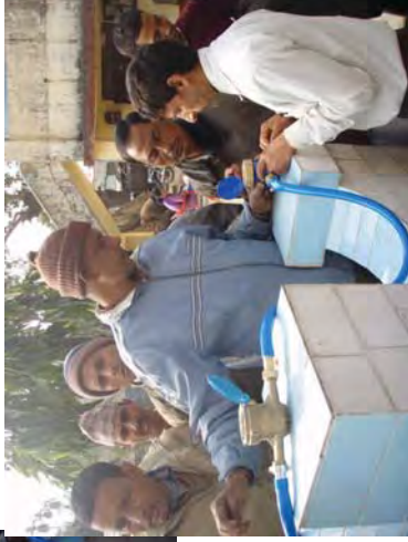
Checking if any leakage at the connection points
