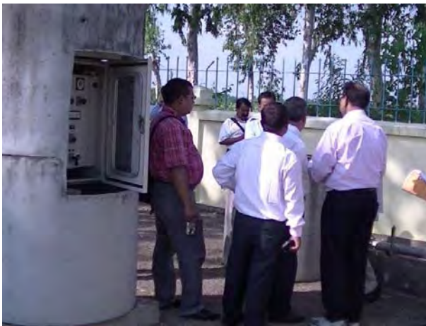
Photo-10 Third country Training in SRWSA in Cambodia Site Visit of Intake Facility Lectured about Monitoring System of Intake Facility at the sites
