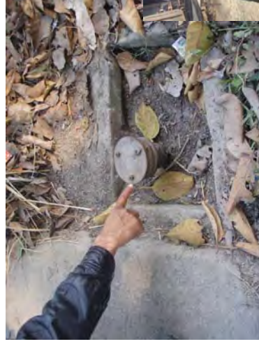
Air valve chamber without cover
