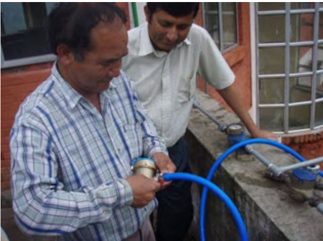
Connecting the water meter
