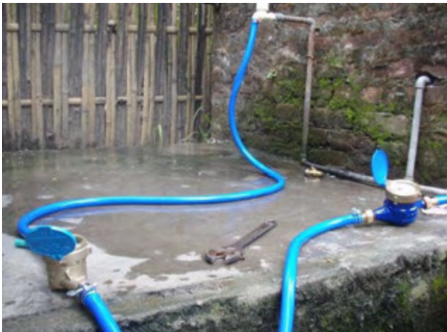
Examination of the existing water meter at the customer's house
