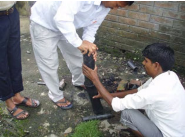
Dhulabari WUSC staff trying to make the handmade socket type conjugation tube.
