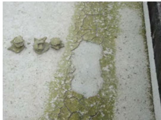
(10) Dried sand to be washed at one of four slow sand filter ponds at Dhulabari WUSC
