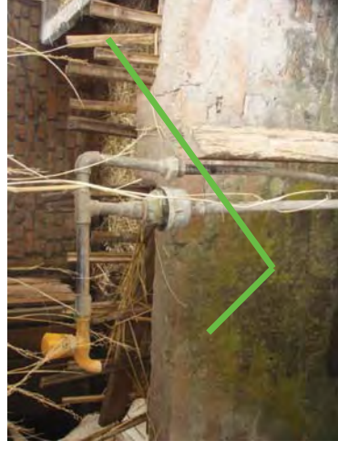
Vertical Type Meter (Correct Installation)
