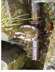
Leakage from washout valve Need to fix and save water
