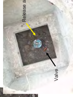
Air valve box cover by concrete (VR-9)
