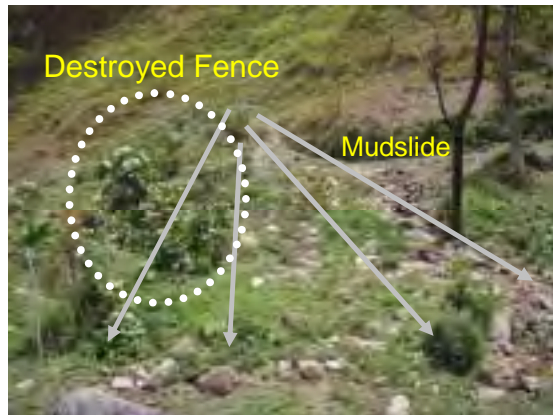
Catchment Area in Intake (May 2010)
