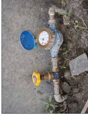
Installed water meter
