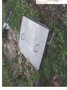
Air valve box cover by concrete (VR-9)
