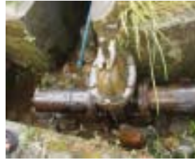
Leakage from washout valve Need to fix and save water
