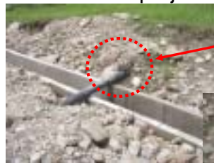
Disconnected pipe
