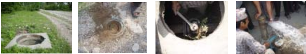
Exploratory investigation of Pipeline Rout
