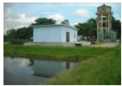
Iron-removal plant at Gauradaha
