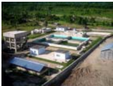
WTP at Dhulabari
