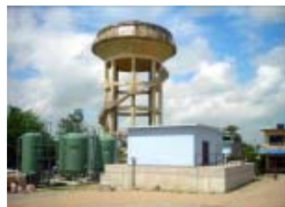
Iron-removal plant at Mangadh
