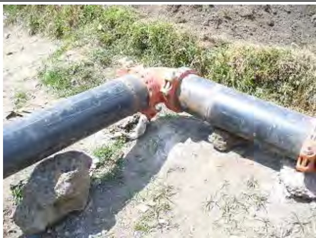
Pipe in the air, support needed
