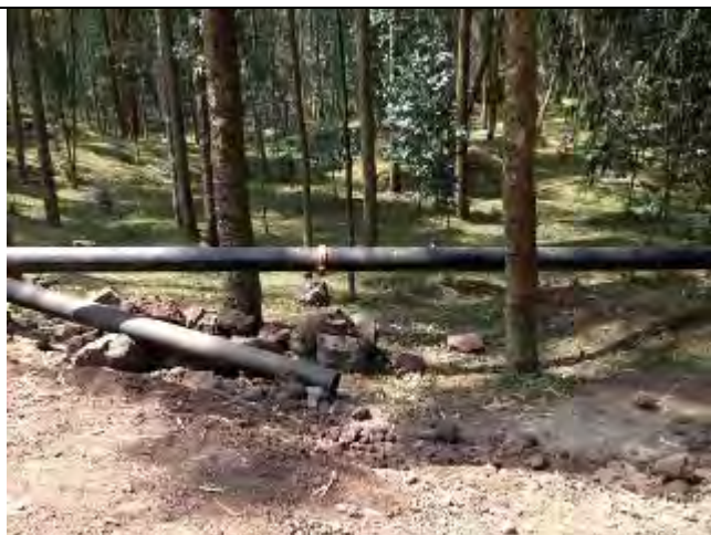
Pipe in the air, support needed
