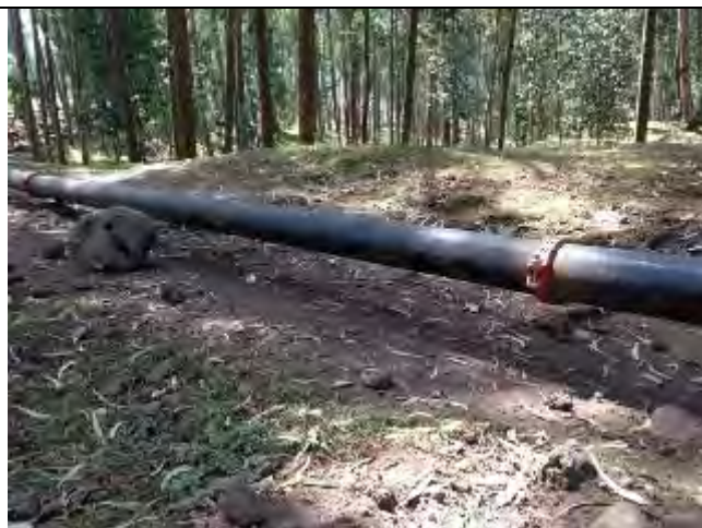
Pipe in the air, supports recommended.
