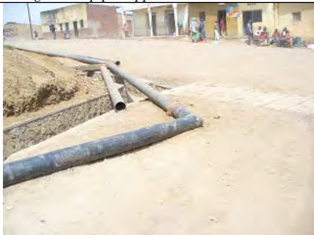
Sharp angle bend; recommended to be exchanged with a long elbow.
