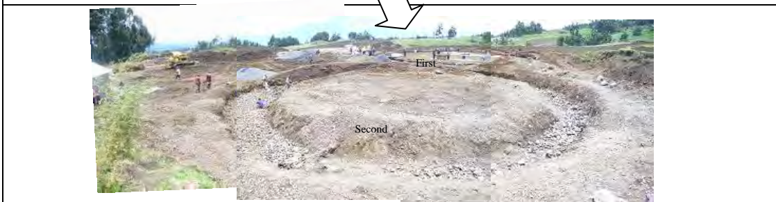
Three water tanks (4,000 m 3 each) were being constructed. Basement re-barring for the first (the above two picture), gravel placing for the second, excavation for the others were conducted.
