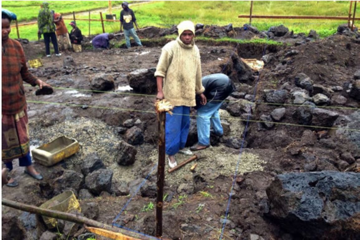
Figure 3 Water intake pump station construction, foundation preparations.
