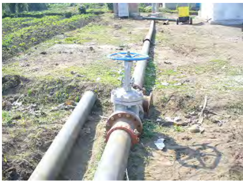
Valve arrangement at the booster pump station
