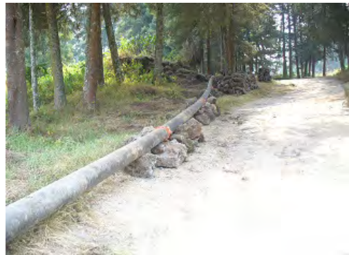
Delivery pipe near Karago Lake (8")
