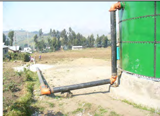
Pipe arrangement to the tank at the booster pump station
