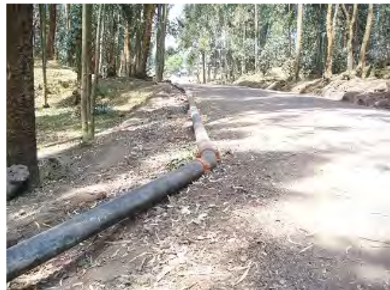
Pipe arrangement along a rural road
