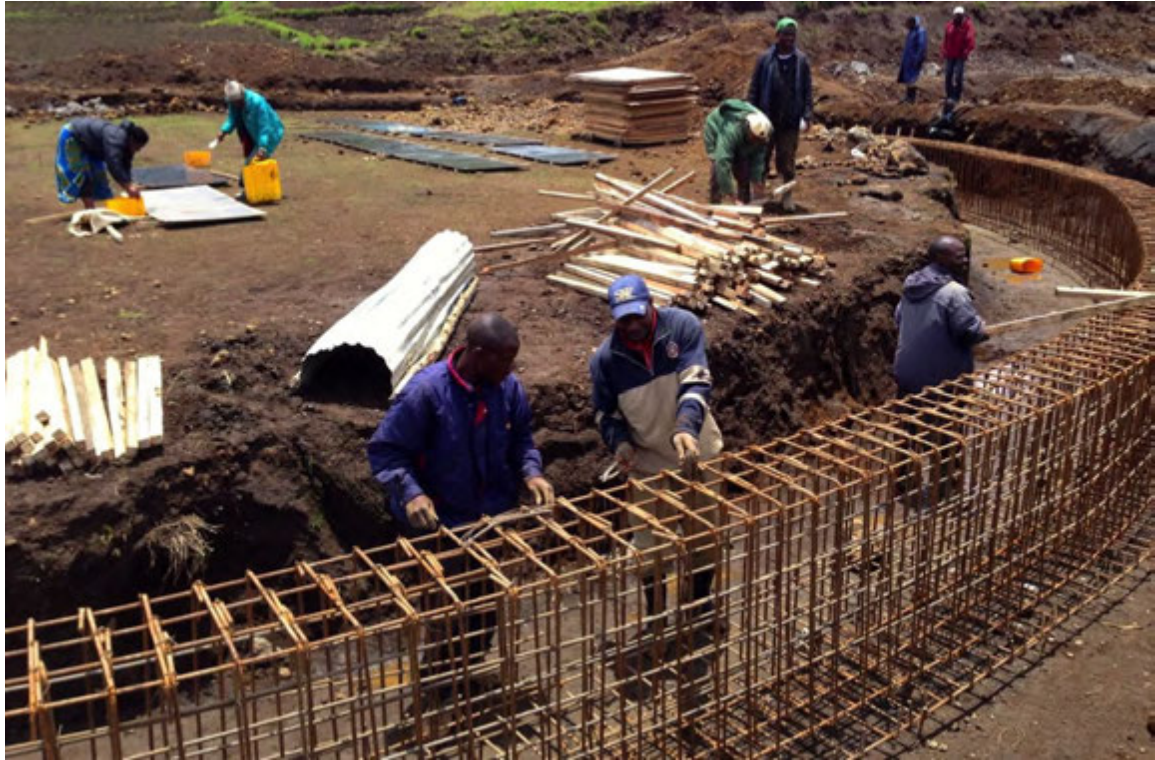
Figure 5 Water tank construction
