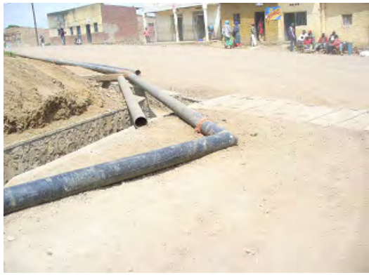
Pipe arrangement at a bend point
