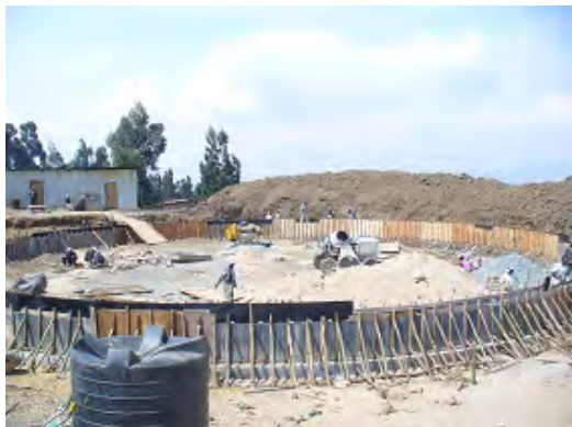
Tank No.3 under construction
