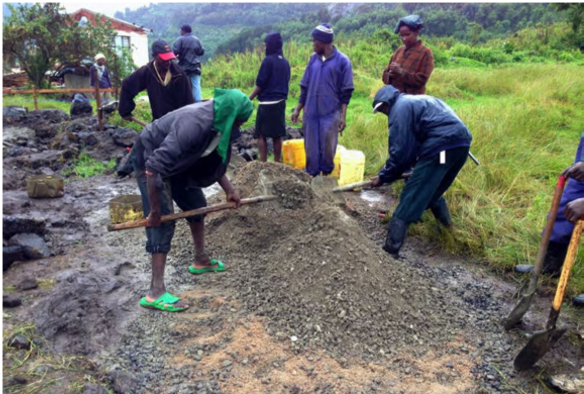
Figure 4 Water intake pump station construction, cement slurry mixing.
