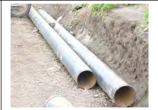
Water supply for the Karisimbi drilling site: Six inches, steel pipes were placed along the some 2-3 km stretch of the main road, photos at the junction of the access road.
