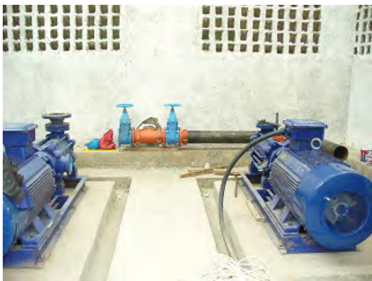
Pump station at Karago Lake ( Q=155\text{m}^3 , V=536\text{m} ) x 2 pumps
