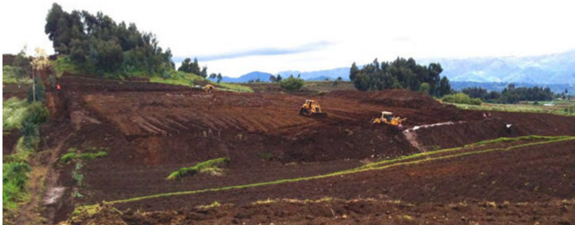
Figure 1 Drilling site construction
