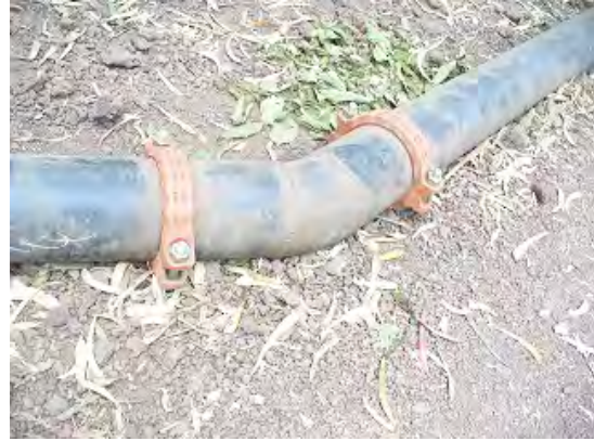
Pipe bend arrangement without pipe support
