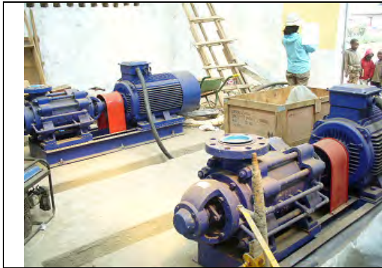
Booster pumps ( Q=155\text{m}^3 , H=268\text{m} ) x 2 pumps
