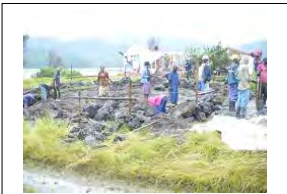
Construction of the pump house at the intake near Kargo lake. Placement of foundation was under way.
