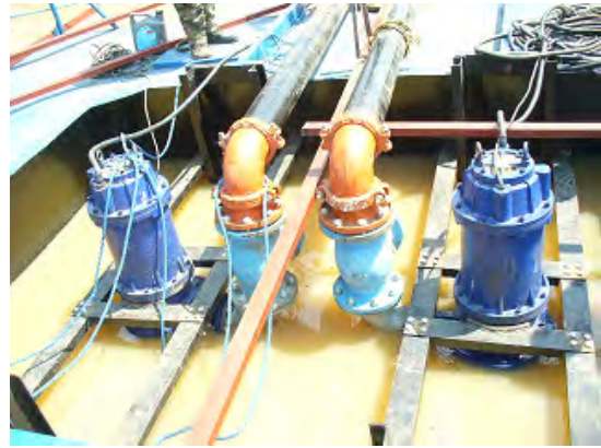
Submersible pumps at Karago Lake ( Q=150\text{m}^3 , H=25\text{m} ) x 2 pumps
