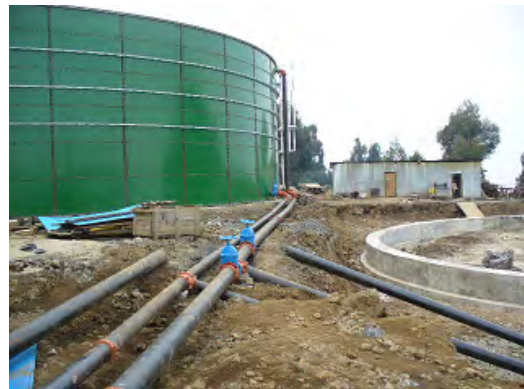
Pipe lines around tanks
