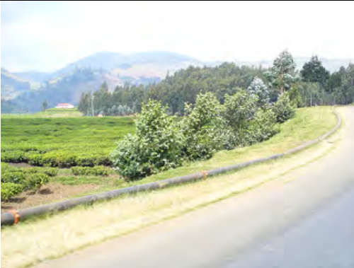
Pipe arrangement along a main road
