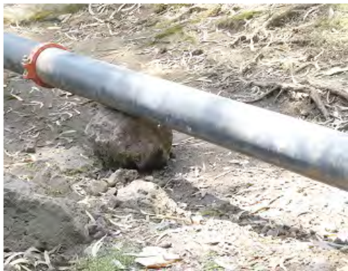
Pipe on a rock support
