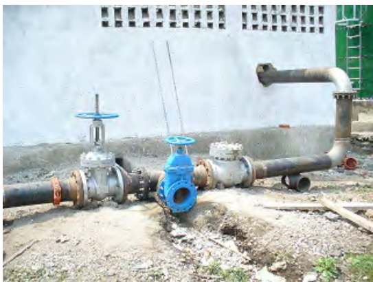
Valve arrangement at Karago lake pump station
