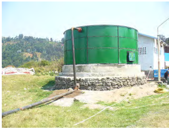
Pump Station at Karago Lake
