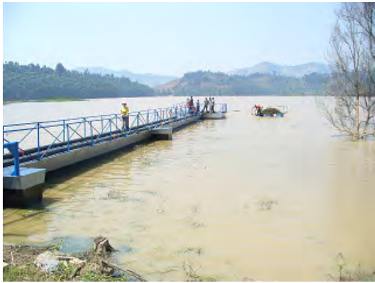
Water intake at Karago Lake
