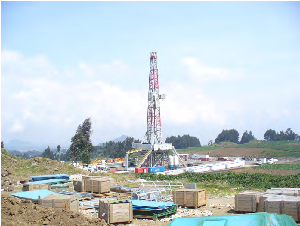
General View of the Drilling Site
