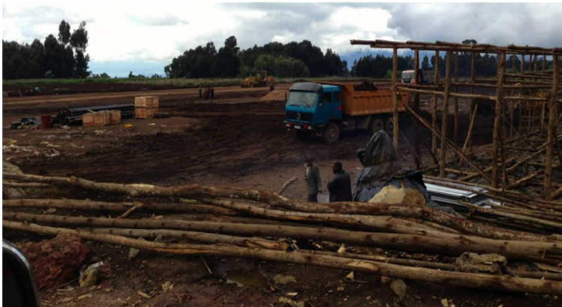
Figure 2 Camp site construction
