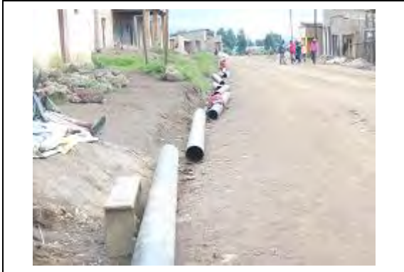
Water supply for the Karisimbi drilling site: Six inches, steel pipes were placed along the some 2-3 km stretch of the main road, photos at the junction of the access road.
