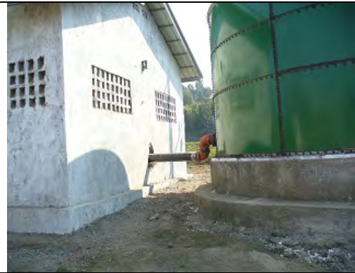
Booster pump station
