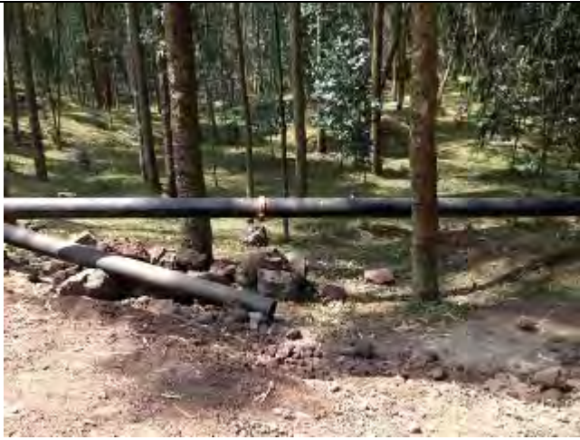
Pipe in the air, support needed
