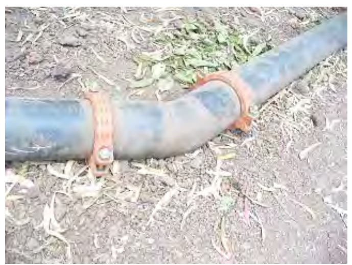
A bent pipe support recommended.
