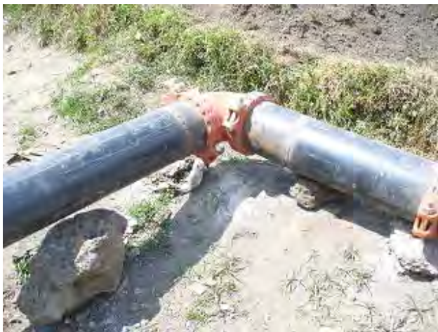
Pipe in the air, support needed
