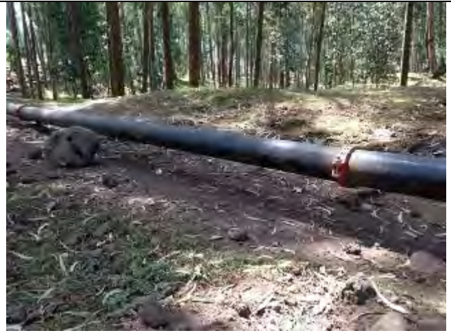
Pipe in the air, supports recommended.
