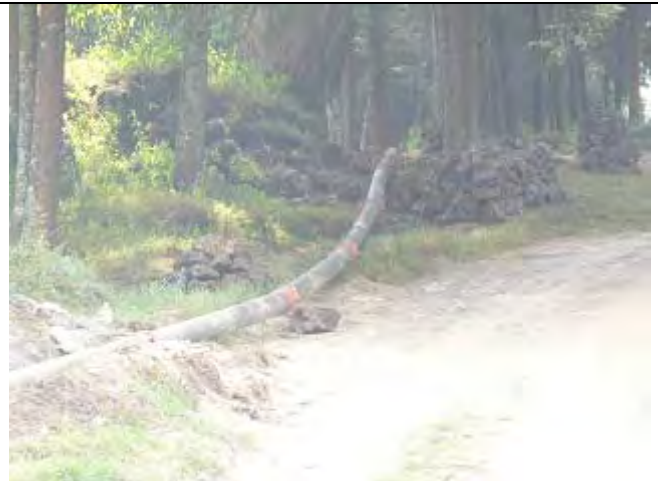
Pipe line in the air at Lake Karago; proper pipe support recommended. Approx 30 MPa internal pressure or more.
