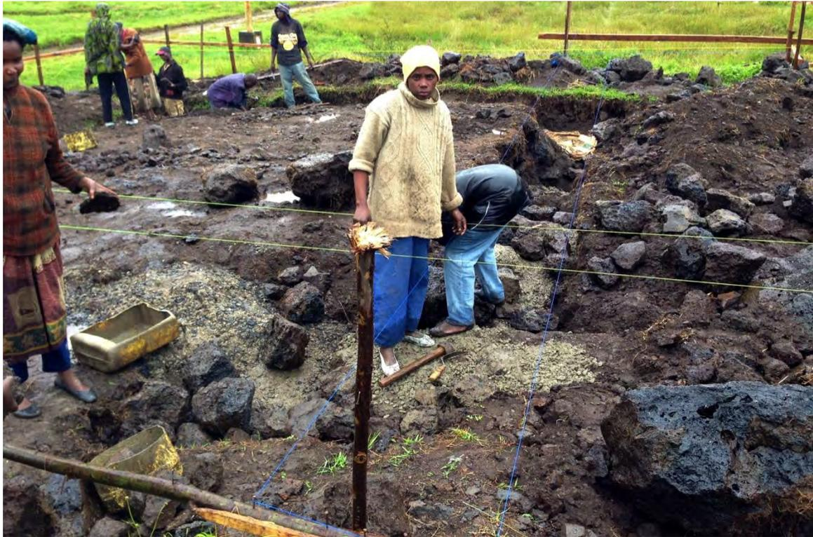
Figure 3 Water intake pump station construction, foundation preparations.
