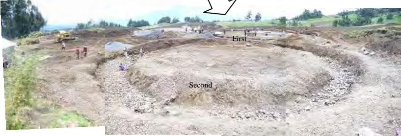
Three water tanks (4,000 m<sup>3</sup> each) were being constructed. Basement re-barring for the first (the above two picture), gravel placing for the second, excavation for the others were conducted.
