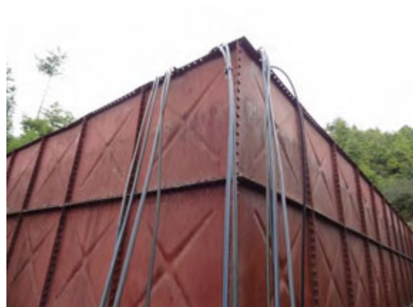
Pipes for drinking water
