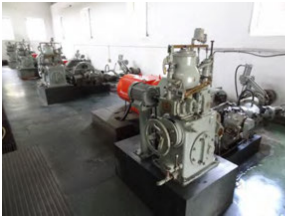
Turbine and Generator
