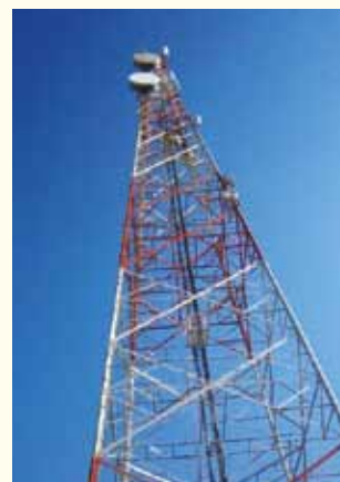
A Tower for Telecommunication in Yangon
