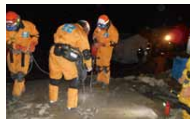
Comprehensive exercise continues around the clock as - Rescue team members break through concrete to reach victim.
