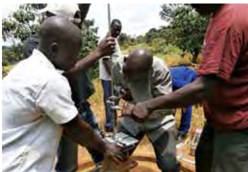
Mechanics learn how to repair hand pumps used to supply water. (Uganda)
