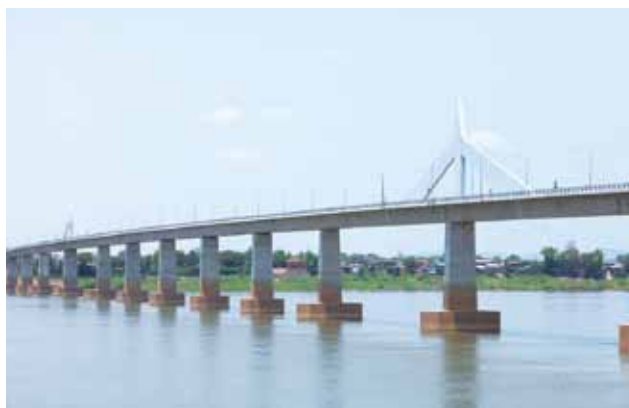
The Second Mekong International Bridge, which links Thailand and Lao, was financed by an ODA loan. The project is part of the construction of an east-west corridor that will extend from Vietnam to Myanmar.
