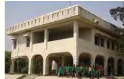
The above school in Bangladesh is an example of mainstreaming DRR. The school was built to also function as an emergency shelter in the case of a disaster.
