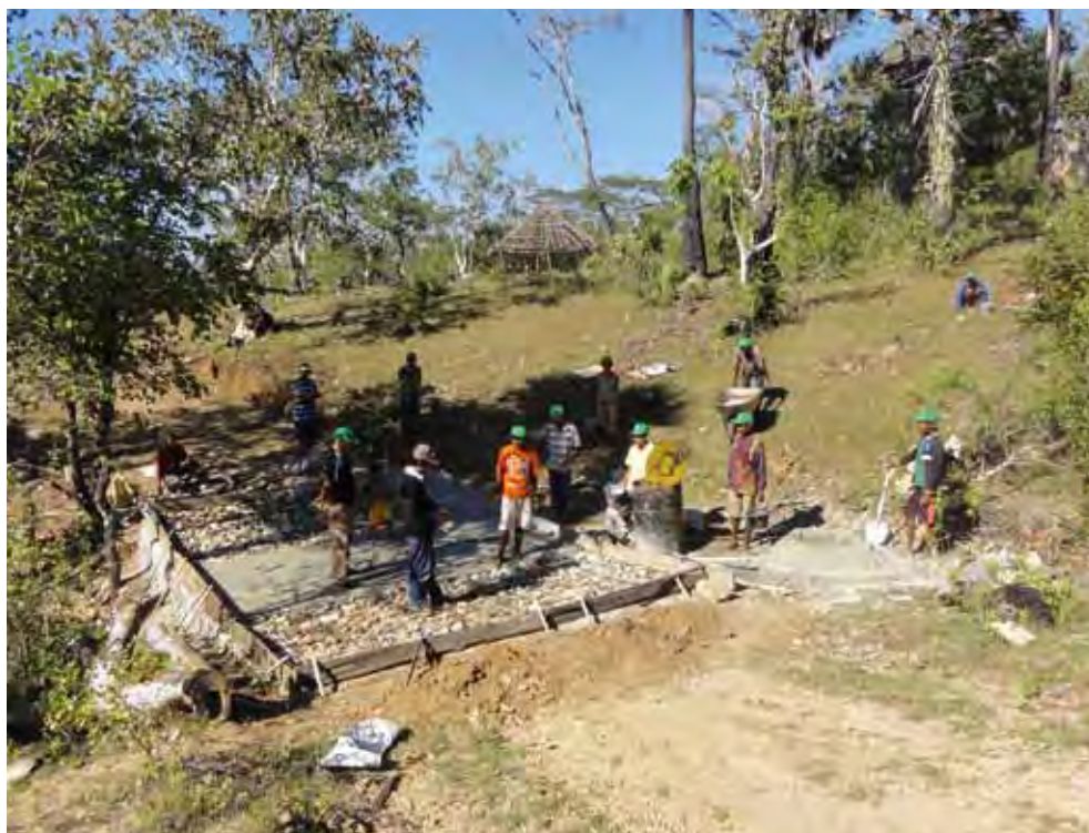
Residents build a community road (Timor-Leste)
