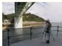
KUMONOS is being used to remotely measure cracks and fissures in a bridge. (Kansai Construction Survey Co., Ltd.)
