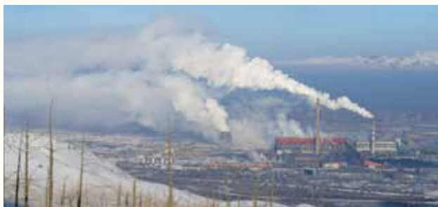
Black smoke being emitted by electric power station
