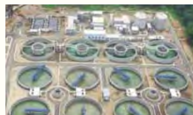
The completed sewage treatment plant
