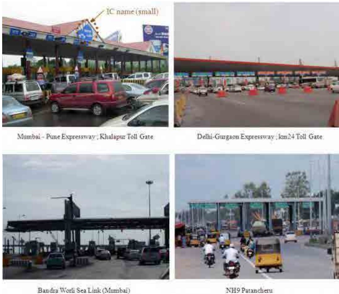
Figure 11.42 Toll Plazas in India
