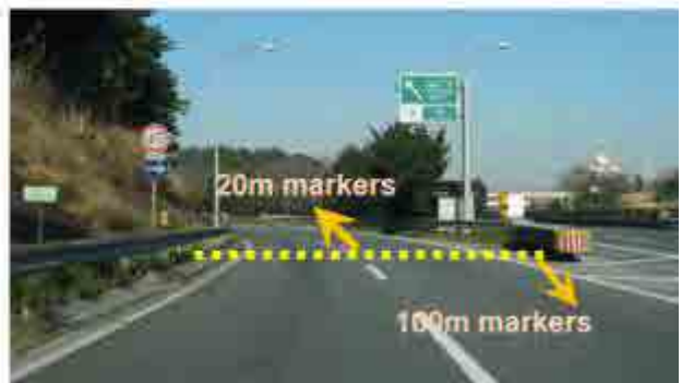
Figure 11.59: Examples of installation of distance markers in Japan
