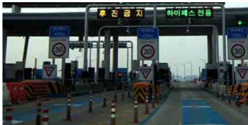
Example in Korea (Incheon Bridge)
