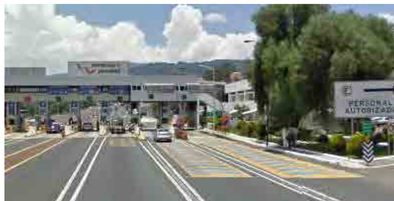
Example in Mexico (Mexico City - Cuernavaca Expressway)
