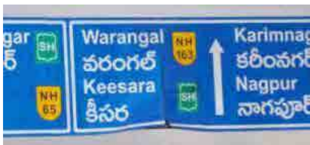
A sign damaged by a vehicle higher than the height limit
