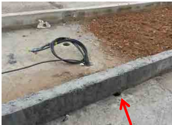
Cable duct found outside of island
