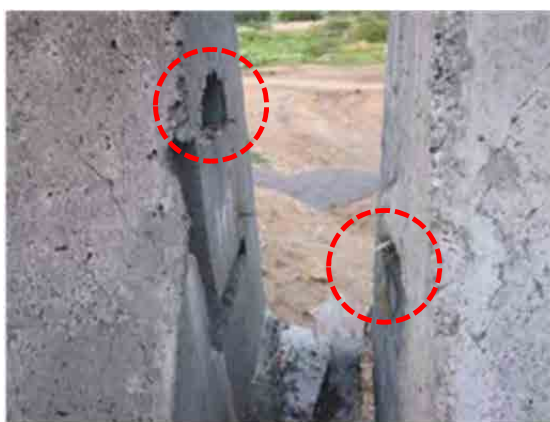
Ducts at different level and duct half covered with concrete (left)
