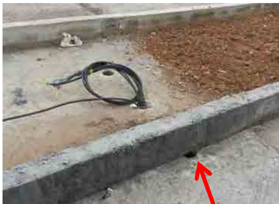
Cable duct found outside of island
