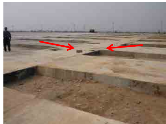
Toll lane not levelled and inclined toward booth
