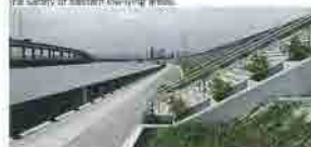
Earthquake-Proof Levee (Nakagawa River, Edogawa Ward)
