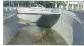
Revetment work (Sagami River, Nerima Ward)
