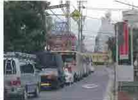
Before removal of rail crossing (near Shūtsu Park (No. 1))
