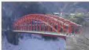
Example of extending bridge operating life (Mitsunashi Bridge, Okazaki town)
