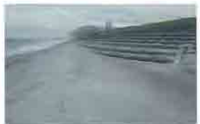
Construction of granite slope retaining (Hatsuda shoreline)
