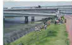
Building Riverside Environments (Nakagawa River, Edogawa Ward)
