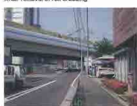
After removal of rail crossing
