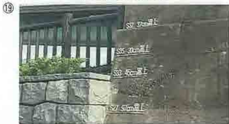
4. Flood control measures Higher revetments
