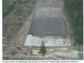
Construction of granite concrete work to prevent landslide...
