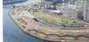
Installed Super Levee (Tonegawa River, Arakawa Ward, Saitama City)
