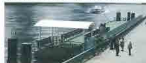
"Tokyo Mizube Line" waterbus and disaster prevention pier (Tonegawa River in Akishita, Chuo Ward)
