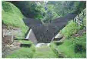
Construction of 1400-ton dam to prevent damage from heavy rain...
