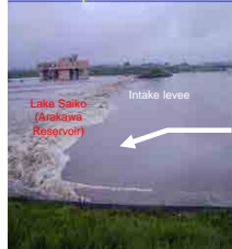
Stormwater flowing into Lake Saiko via an intake levee located at the lake's upstream section
