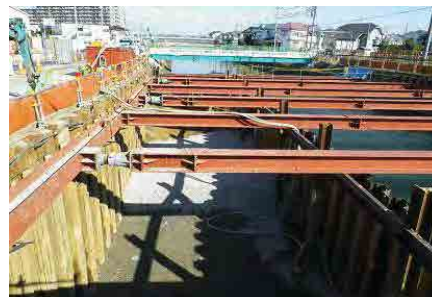
Construction work in a residential area (provision of a school road)
