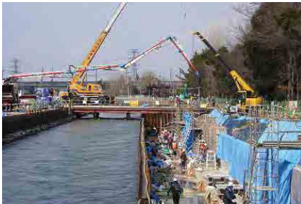
Concrete placement by a concrete pump
