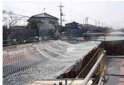
Construction work in a residential area (permanent provision of acoustic barriers)
