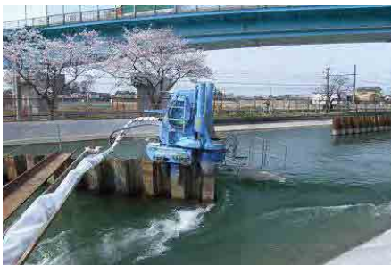
Construction work for oil protection above the water
