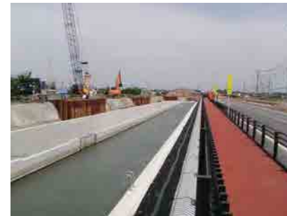
Construction of the administrative road
