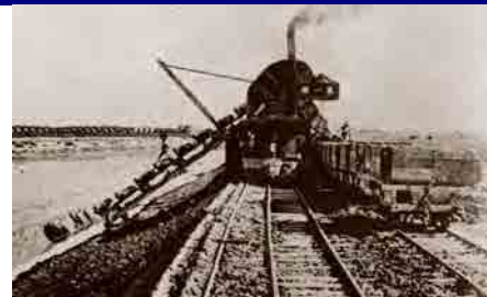
2. A channel was excavated using a steam excavator.
