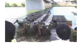
▲ Connecting boats for transporting heavy machinery
