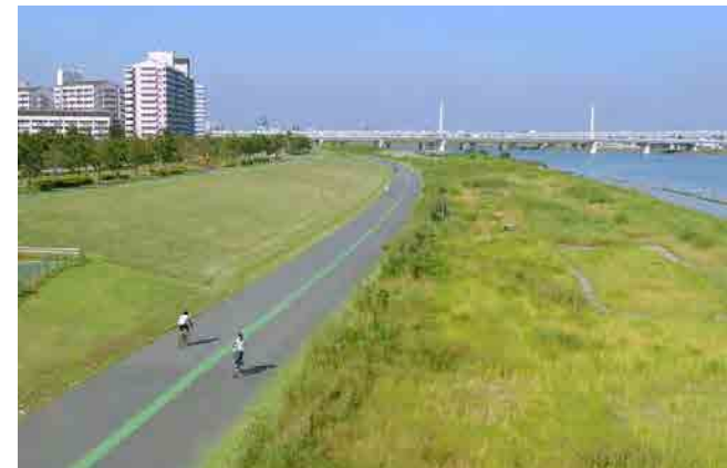
The Tokyo leg is completed. 57.0-km (98%) of the 58.2 km road has been constructed. The remaining 1.2-km section will be constructed on the river's left bank in Kawaguchi City, Saitama Prefecture in step with construction of the super levee project.
