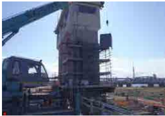
Reinforcing a river structure against bending and shear failure (Steel-plate lining)
