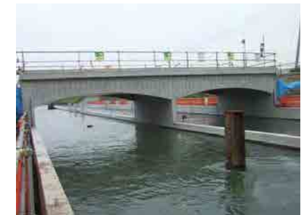
Water passing along both sides of the banks (under the bridge)
