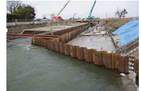
Construction work with excavated surfaces being protected
