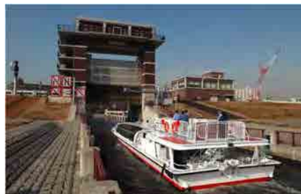
Front lock gate
