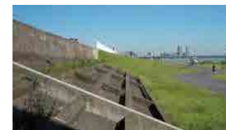
Arakawa River's storm surge barrier
