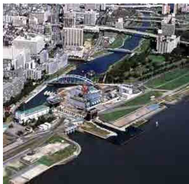
Aerial view of the Arakawa Lock Gates
